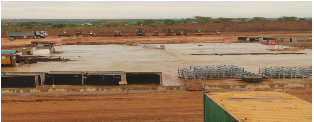
Figure 11: Site preparation for drilling at JBR10
