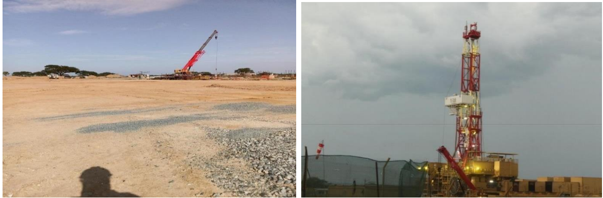
Figure 8: Variation of activities at JBR9 (well pad preparation and rig setup)
