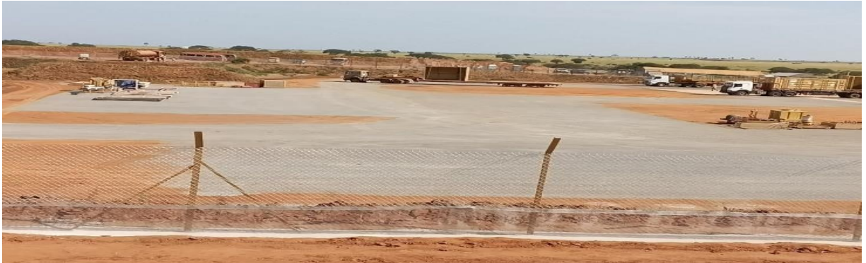
Figure 6: Well pad preparation at JR3
