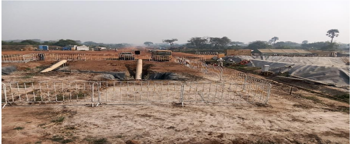
Figure 12: Pipes at the HDD pulled below the Nile River Bed
