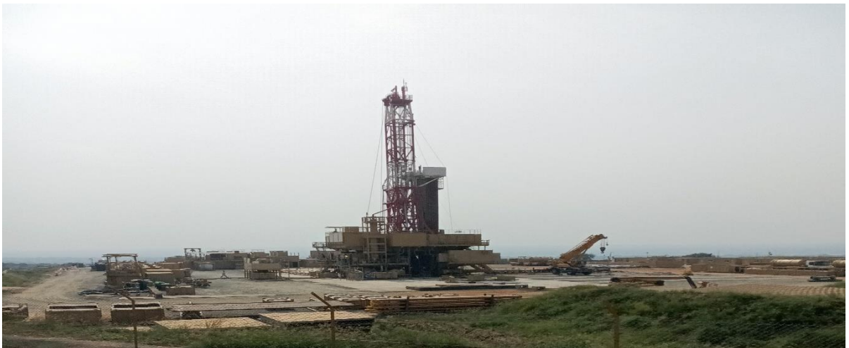
Figure 7: Drilling at JBR2
