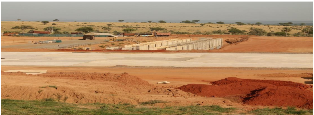
Figure 9: Site preparation for drilling at JBR8
