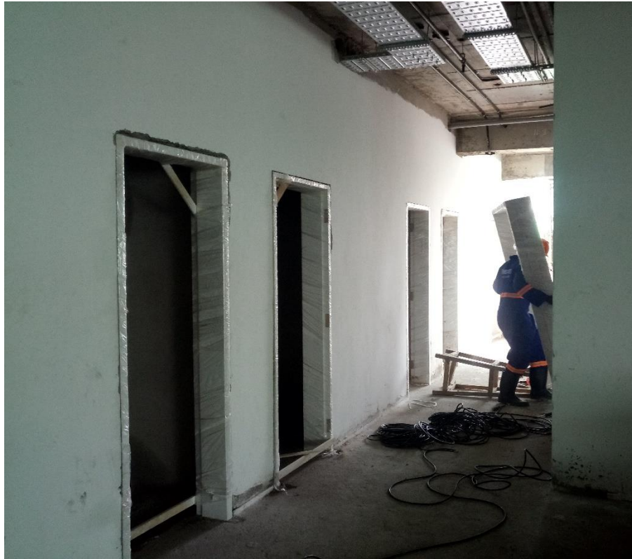
Fig 82; Fixing door frames.
