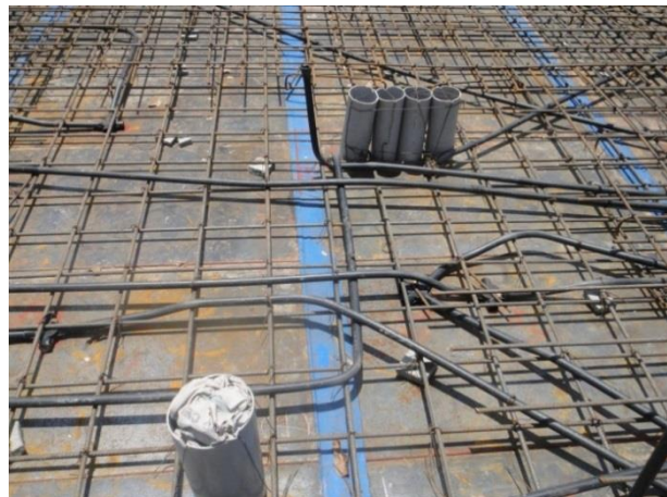
Fig 48; Sleeves and electrical conduits fixed.
