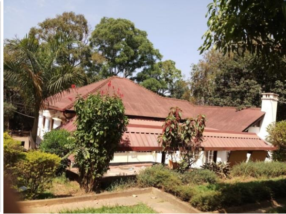
Figure 2: Existing building before development
