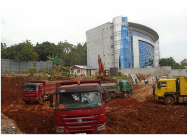
Figure 3: Site excavation to road level.
