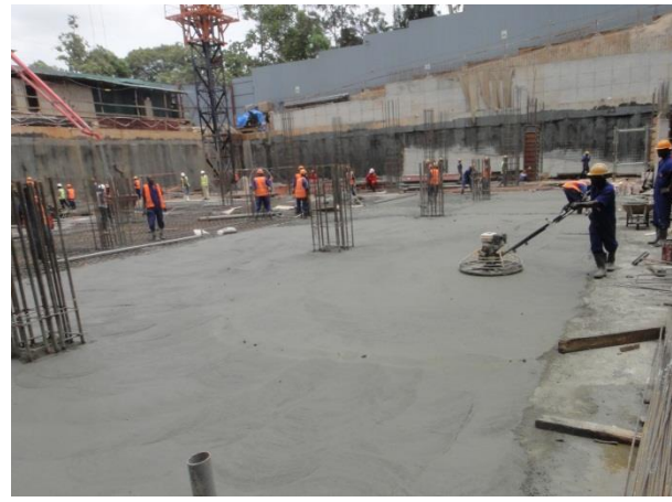
Fig 30; Power floating the concrete surface.
