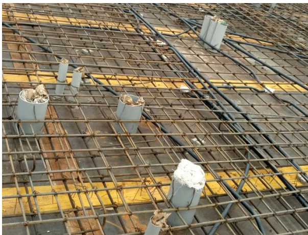
Fig 37; Sleeves and conduits for service fixed.
