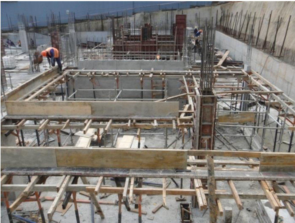
Fig 79; Fixing formwork to beams.
