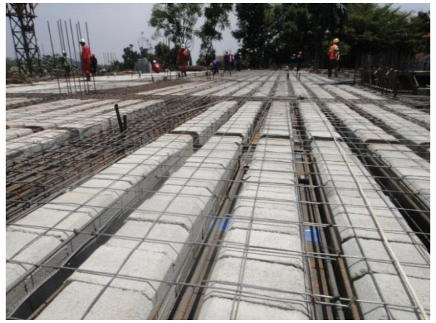
Fig 46; Maxpan blocks laid onto the slab deck.
