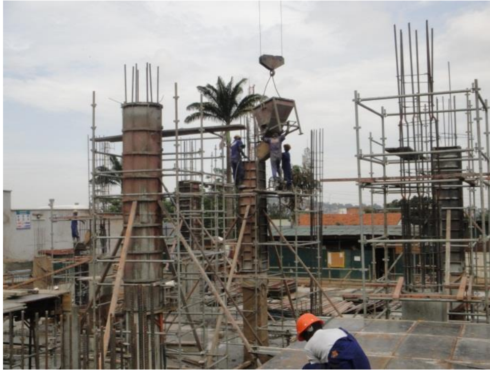
Fig 76; Casting concrete to columns.
