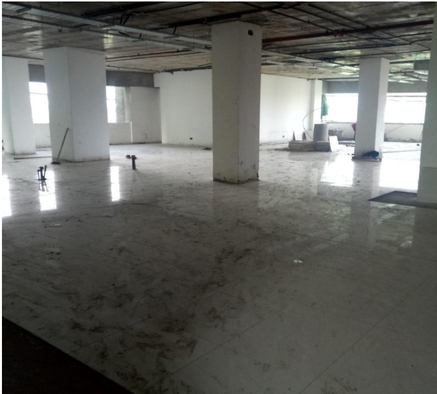
Fig 85; Laying floor tiles.
