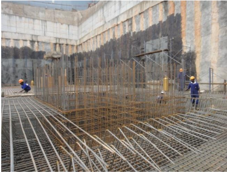
Fig 72; Starter bars for lift shaft walls.
