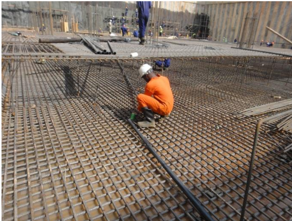
Fig 73; Laying electrical conduits into raft reinforcements.
