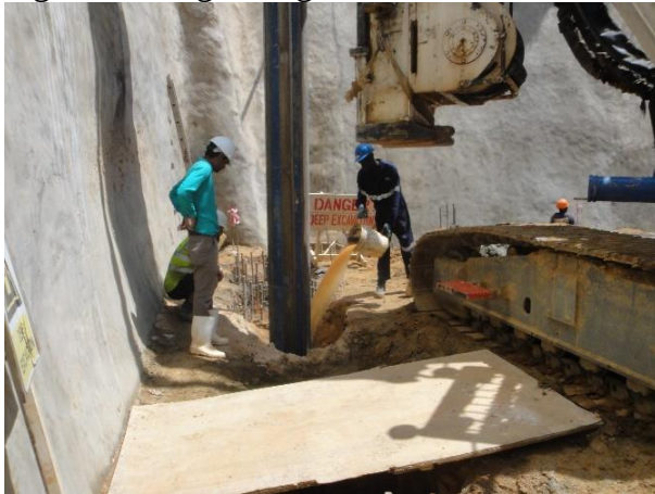
Fig19; Applying water to cool the bucket
