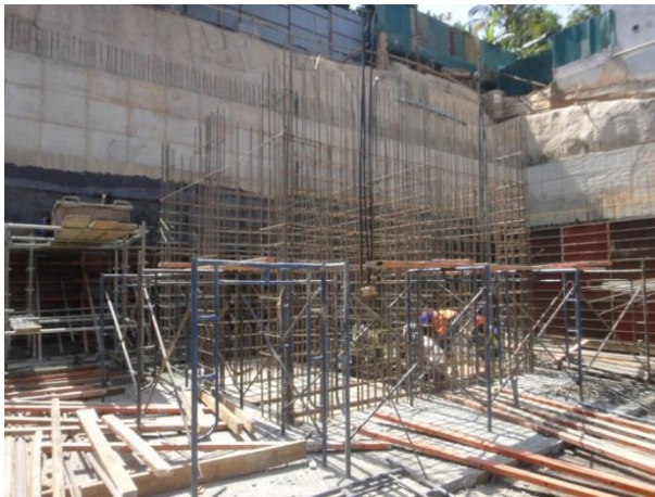
Fig 31; Fixed lift shaft reinforcements.
