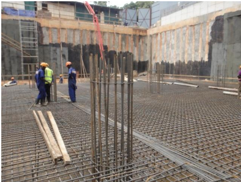
Fig 73; Columns bars fixed onto raft reinforcements.
