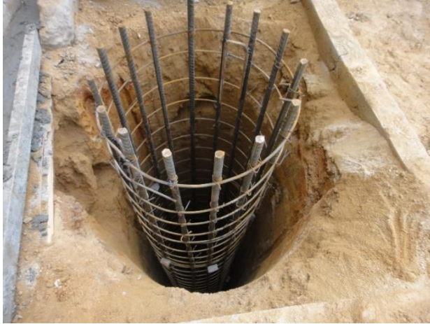
Fig9; Steel cage ready to receive concrete.
