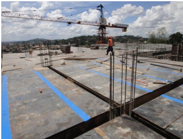
Fig 45; Decking to beams and slab.
