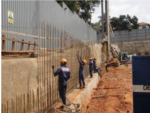
Fig15; Rebar works to the retaining wall.
