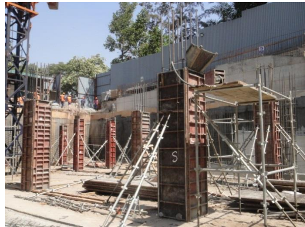
Fig 32; Formwork fixed to columns.
