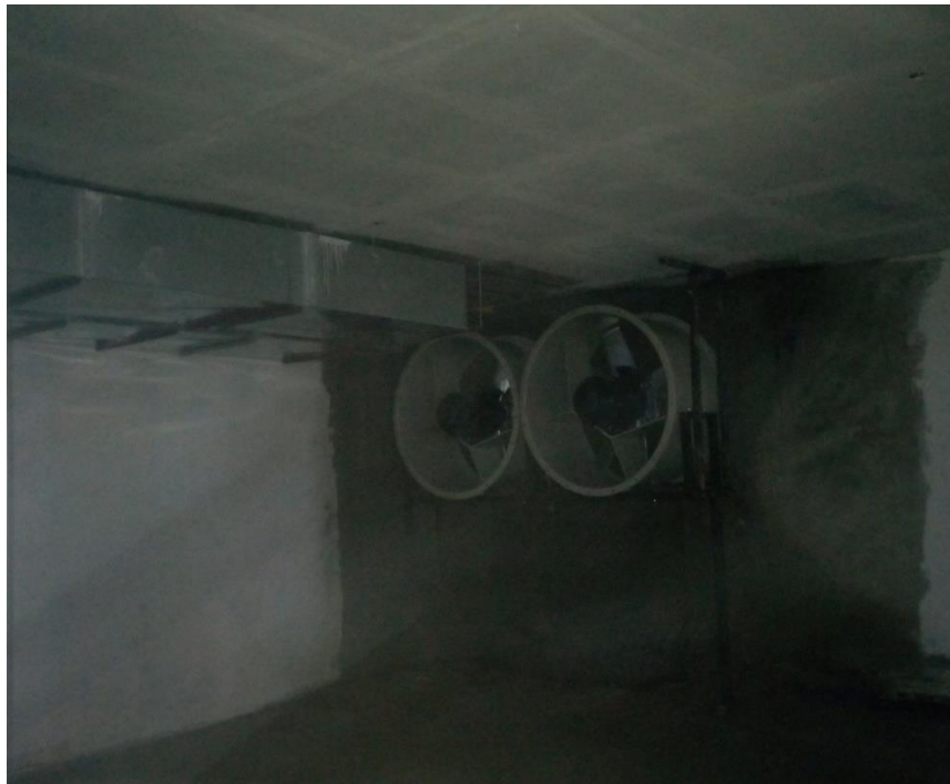
Fig 93; Basement extraction fans fixed.
