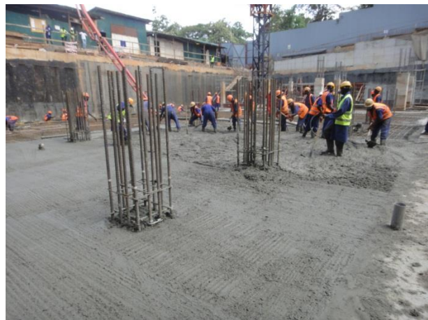
Fig 38; Casting concrete to solid slab.
