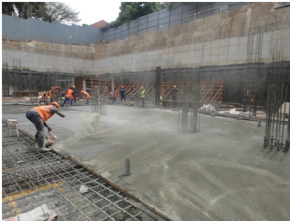
Fig 29; Fosroc Nitro floor hardener applied
