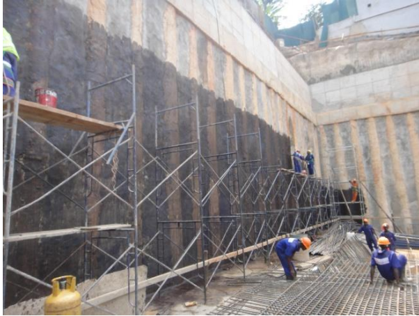
Fig23; Applying water proof primer.
