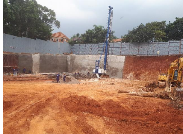
Fig4; short Crete concrete applied to excavations embankments.
