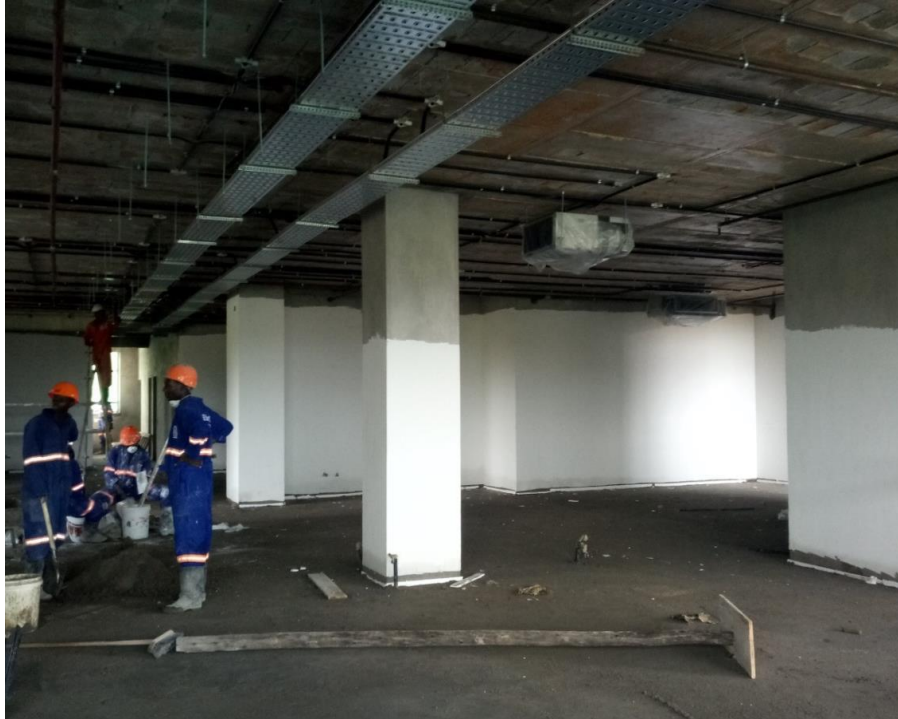
Fig 86; Painting works progressing.
