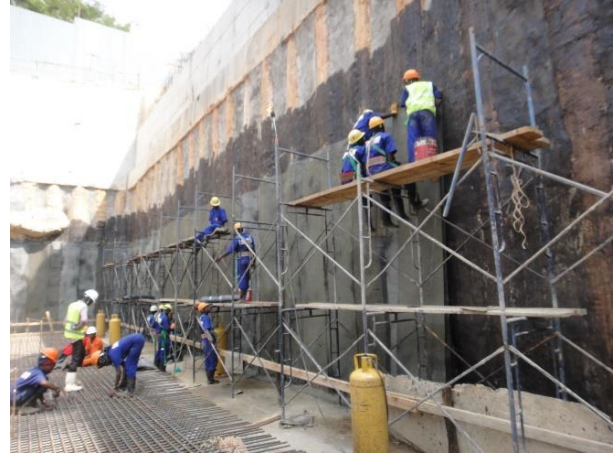
Fig24; Applying the APP membrane.
