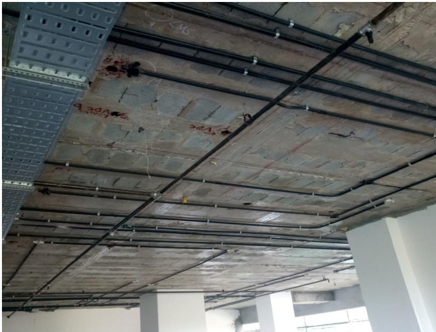
Fig 87; Sprinkler pipes fixed onto the slab soffit.
