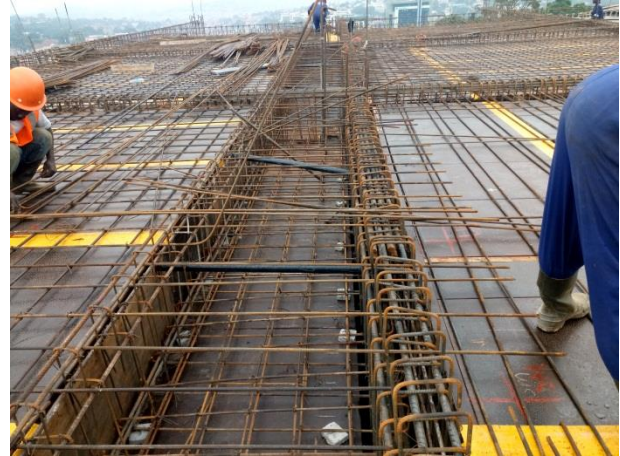
Fig 54; Rebar works to the roof gutter.
