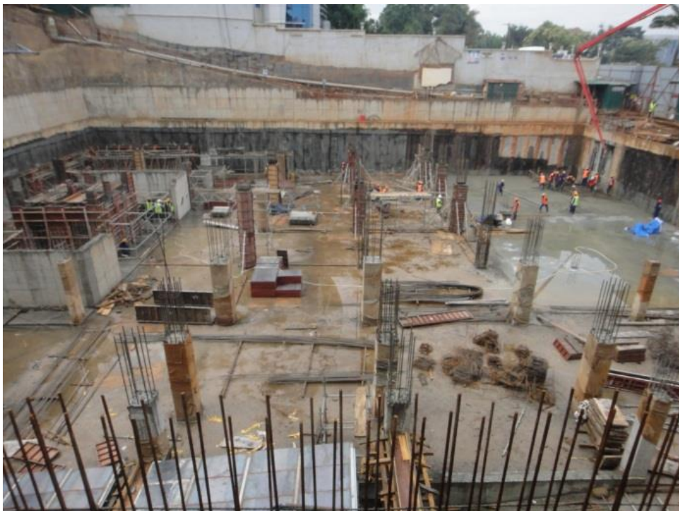
Fig 75; Works in basement3.
