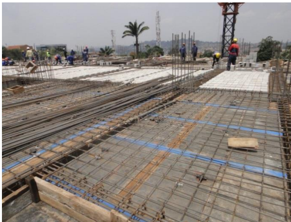
Fig 47; Rebar works to slab.
