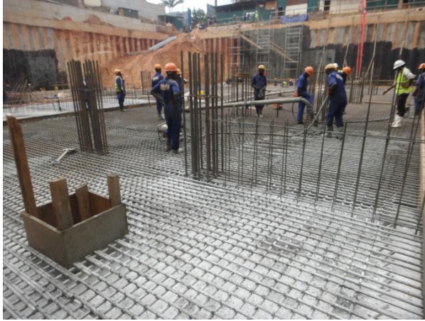
Fig 27; Casting concrete to 800mm depth.
