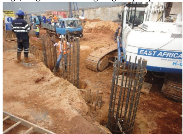
Fig8; Steel cages lowered down into pits.
