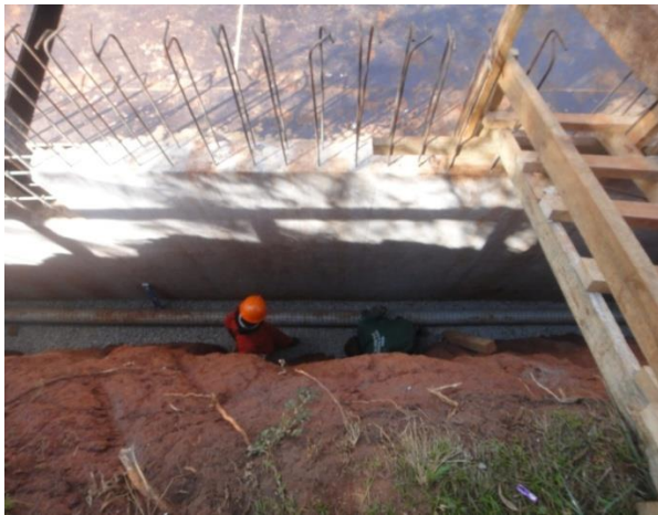
Fig 39; PVC pipe laid onto stone chippings.
