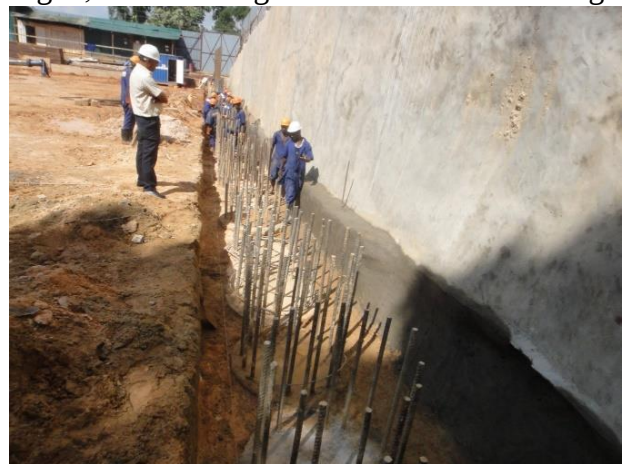
Fig12; Excavating for the pile cap beam.
