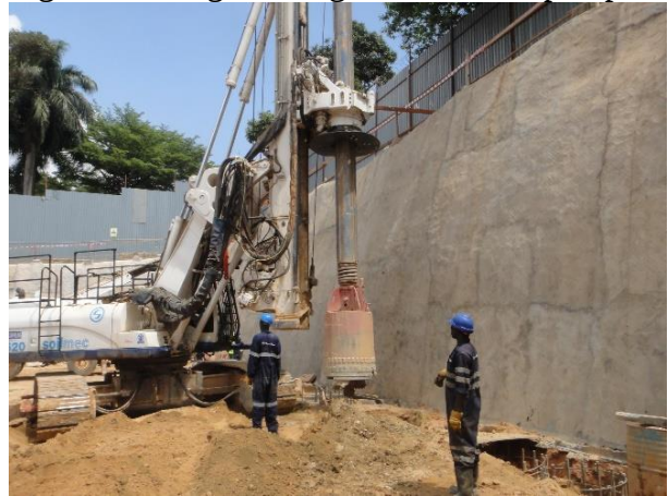
Fig20; Placing the cleaning bucket into the pit.
