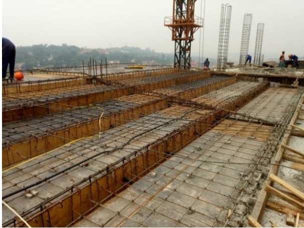
Fig 49; Rebar works to the sitting gallery.
