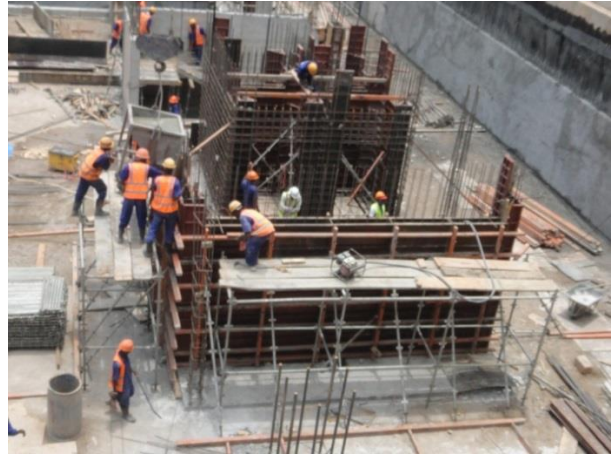
Fig 34; Formwork fixed to shear walls.
