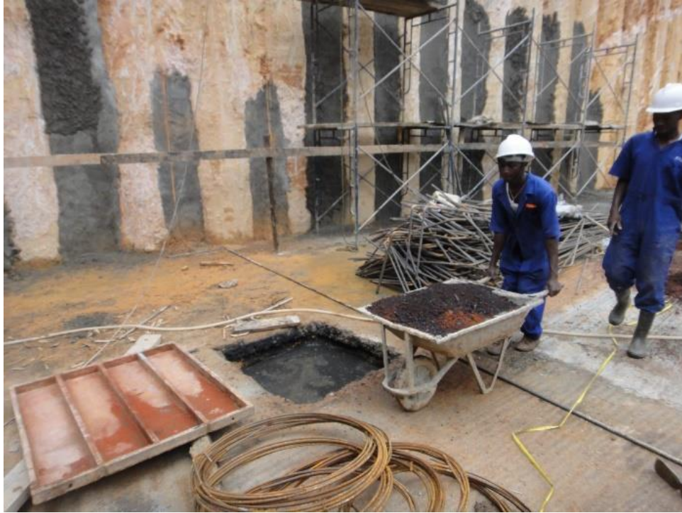
Fig 72; Putting charcoal in earthing pits.
