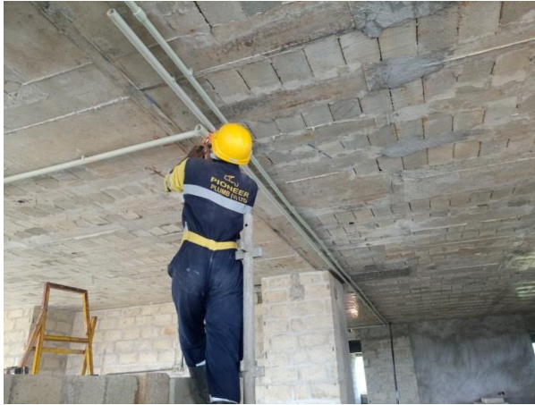
Fig 61; Fixing PPR pipes for fresh water.
