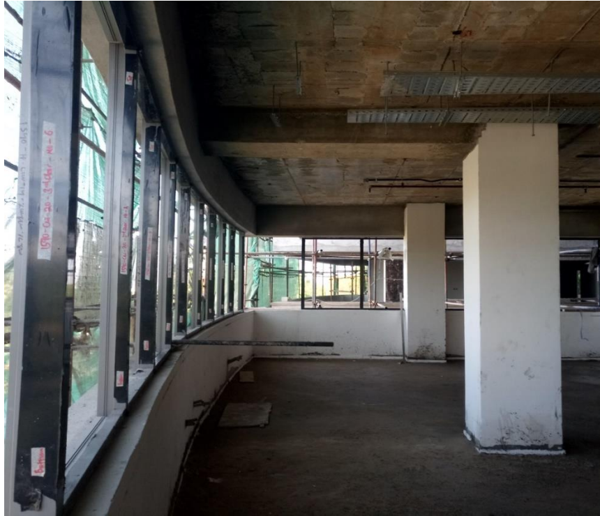
Fig 90; Fixing window aluminium frames.
