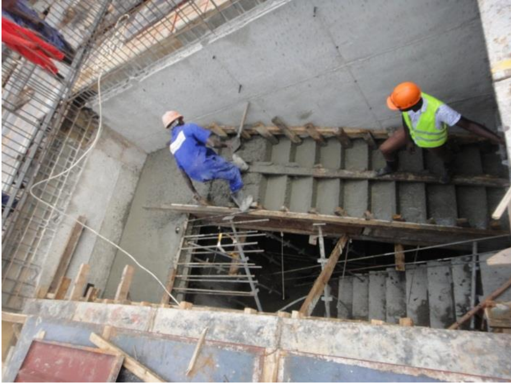
Fig 78; Casting concrete to staircases.
