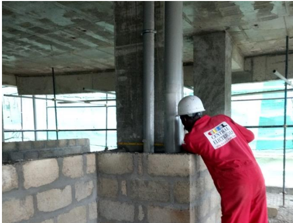
Fig 63; Securing rain water pipes from roof.
