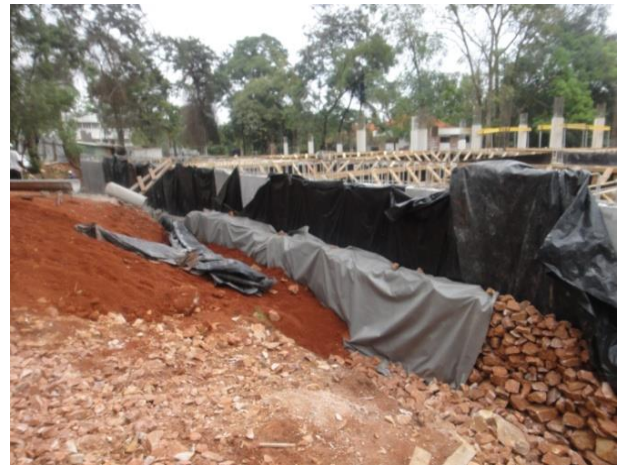
Fig 40; Construction of the dry wall.
