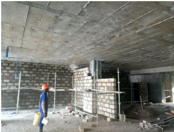
Fig 51; Block walling to office area.
