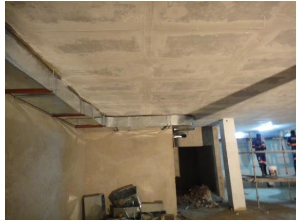
Fig 64; Basement extraction ducts fixed.
