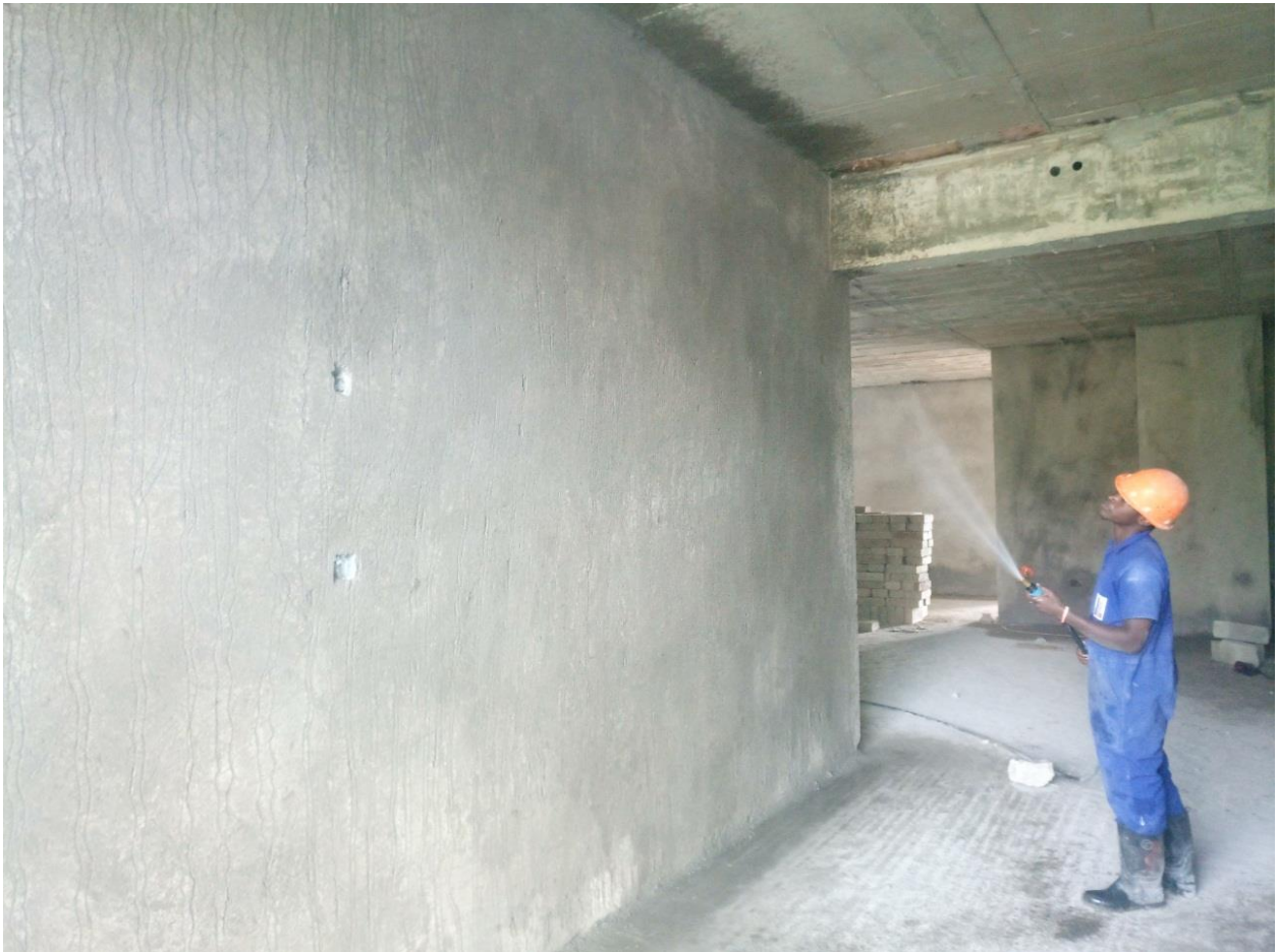
Fig 57; Curing to plaster works.
