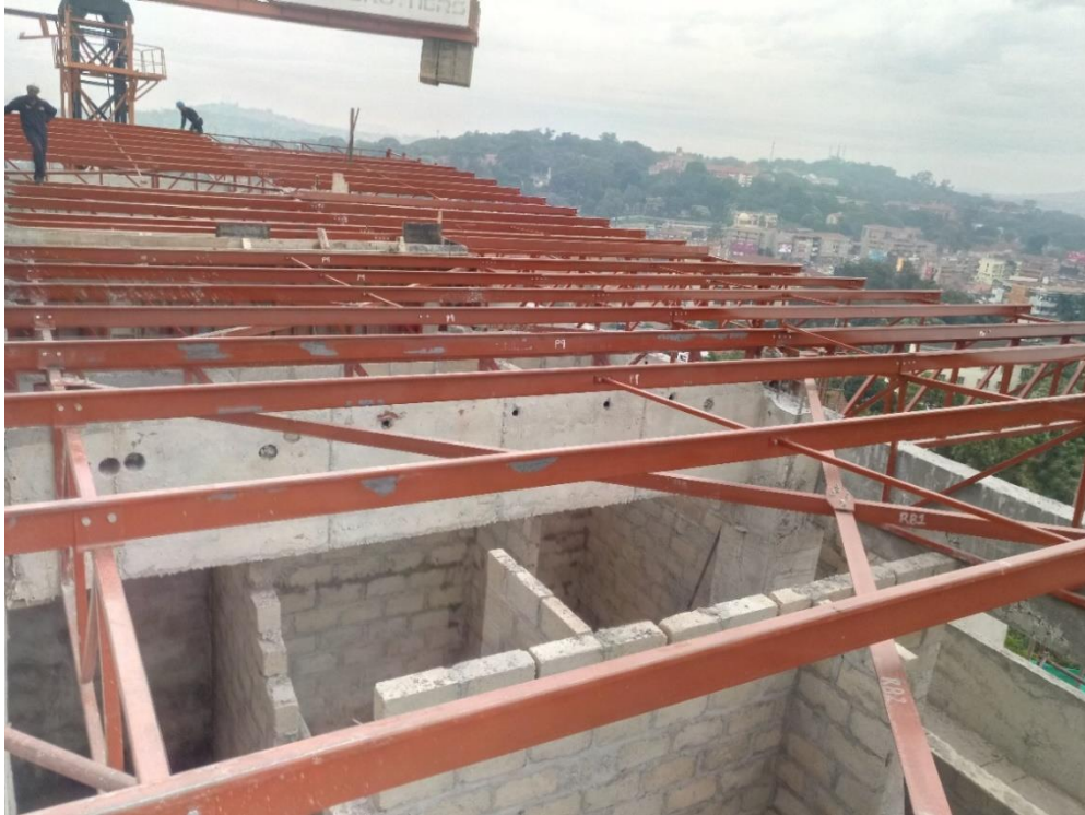
Fig 80; Purlins fixed onto roof girders.
