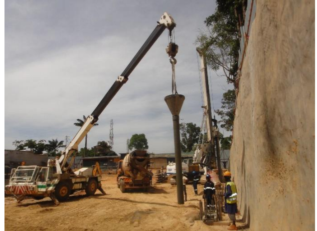
Fig10; Funnel being lowered into the steel cage.
