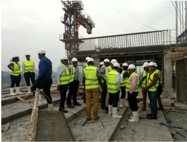
Fig 70; Team conducting site inspection.
