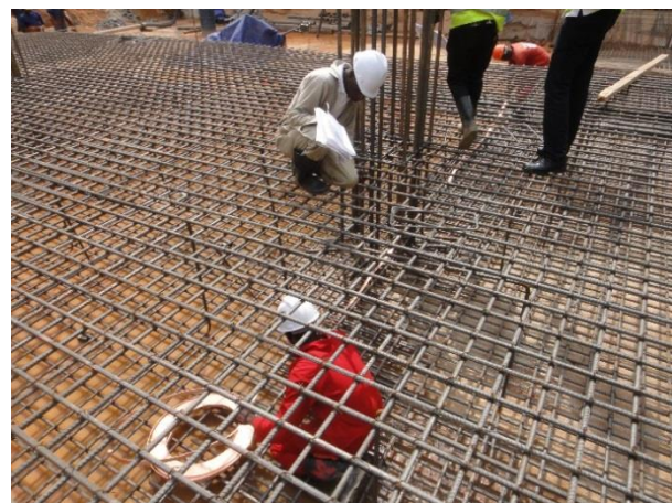
Fig 26; Laying the electrical copper tape.
