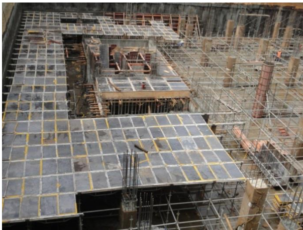
Fig 35; Decking to slab
