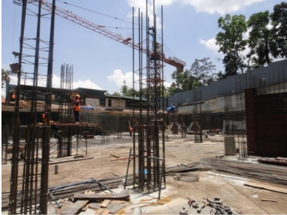
Fig 74; Column reinforcements fixed.
