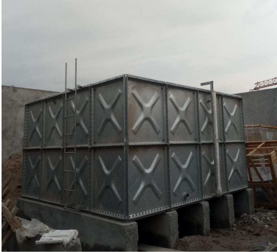
Fig 94; Assembling the water tank at the roof slab.
