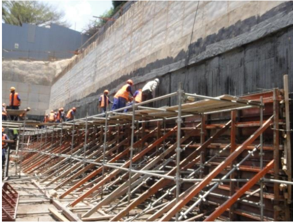
Fig 33; Formwork fixed to retaining walls.
