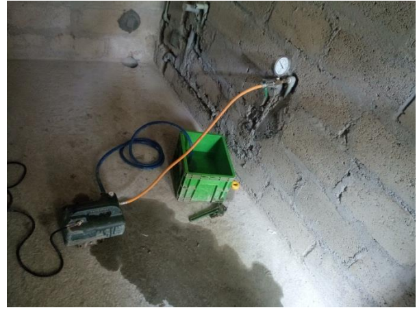
Fig 62; Pressure testing to PPR pipes.
