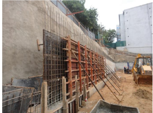
Fig16; Formwork to the retaining wall.
