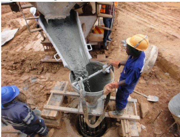
Fig11; Casting concrete to the pile.
