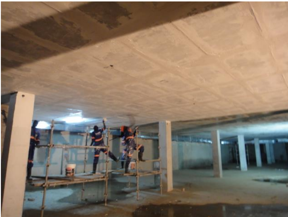
Fig 81; Painting works in basement.
