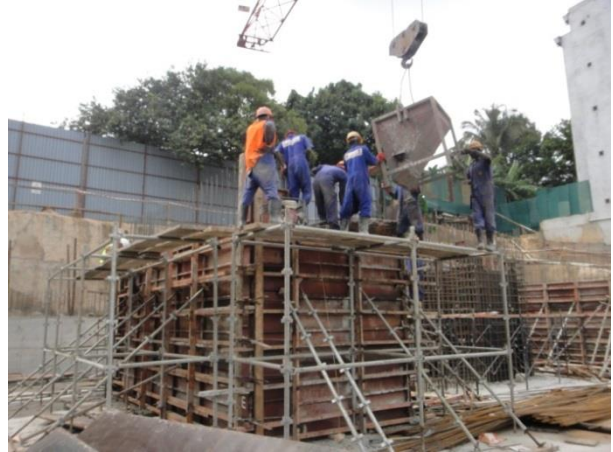
Fig 44; Casting concrete to lift shaft walls.
