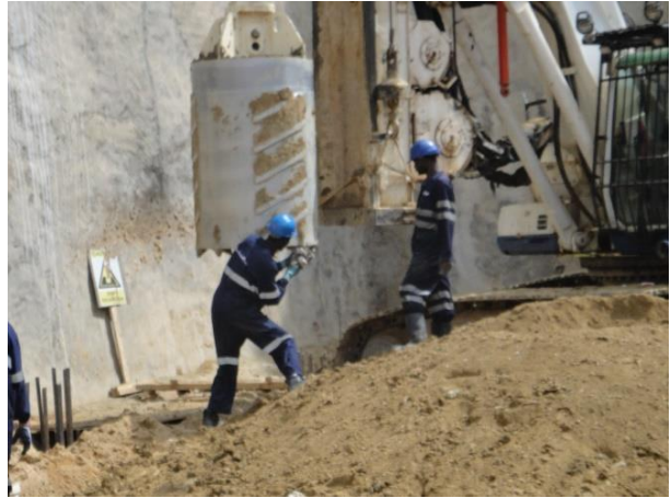
Fig18; Inserting a coring bucket to the pile pit.
