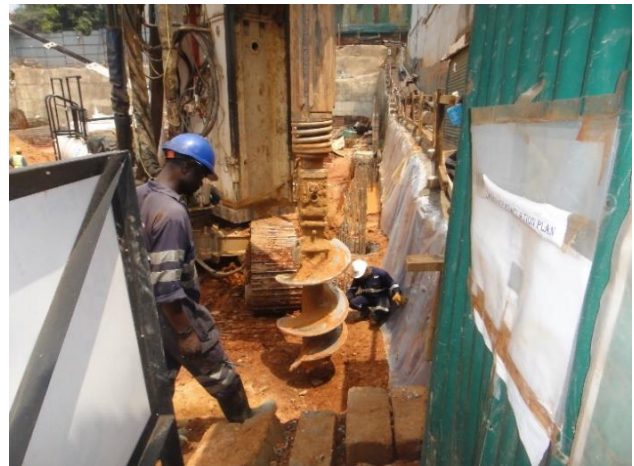
Fig6; Auger machine targeting the pile position.
