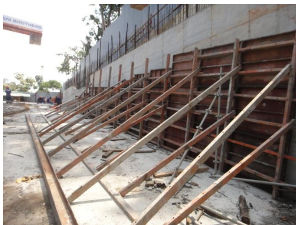
Fig 41; Formwork fixed to retaining wall.
