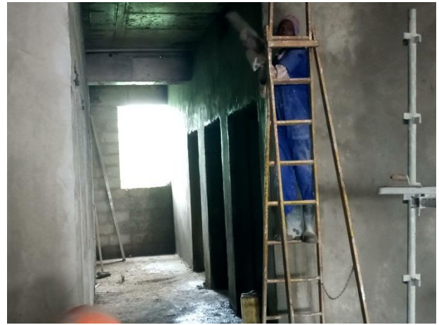
Fig 56; Plastering to walls.
