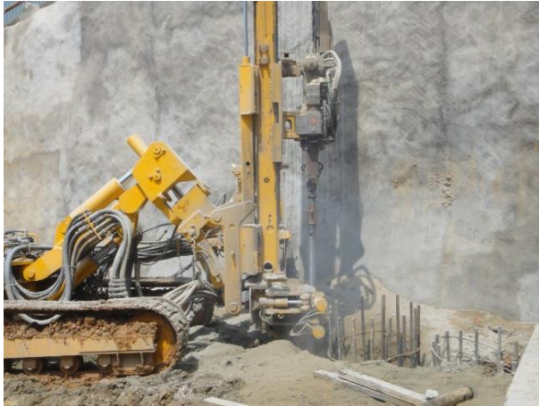
Fig17; Drilling through the rock.
