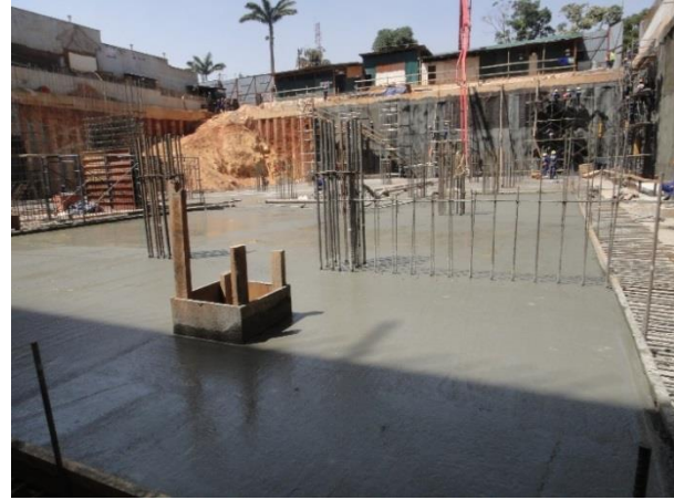
Fig 28; Casting concrete topping of 300mm.
