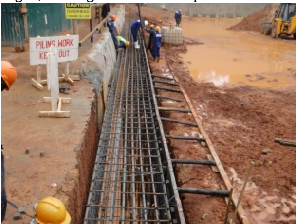
Fig13; Fixing steel and formwork to the pile beam
