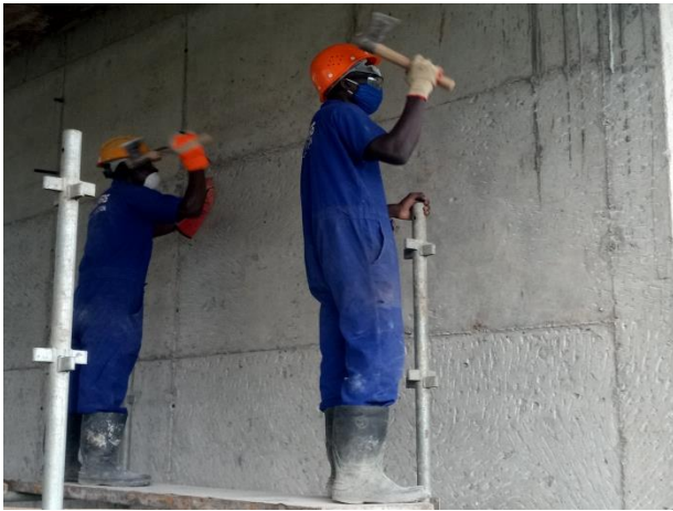
Fig 55; Hacking concrete surfaces.
