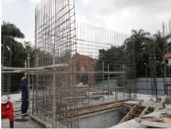
Fig 43; Rebar works to the shear wall.
