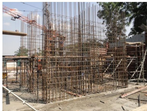
Fig 42; Rebar works to lift shaft walls.
