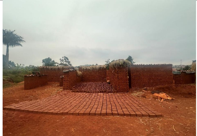
Moulded Mud Bricks Before Stacking
