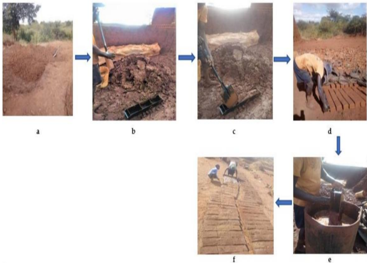
Figure 2.2: Excavation, Preparation and Molding Processes. (a) Excavation of soil with digger and shovel; (b) Covering of the unused mortar portion to prevent evaporation; (c) Filling and levelling of mold content with shovel; (d) Inversion of mold to extrude the content; (e) Washing of mould prior to refilling with mortar; (f) Sequential arrangement of wet bricks for drying and pouring of sand on the wet bricks. (Source; Aniyikaiye et al., 2021)
