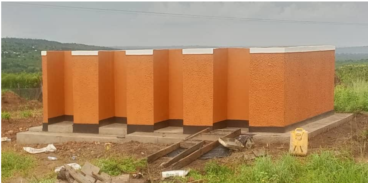
Photograph showing an Eight-unit shower block
