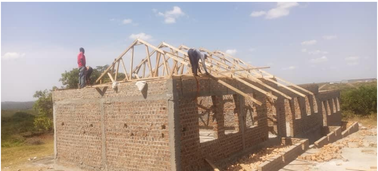
Photograph showing roofing of the one unit three classroom block facility
