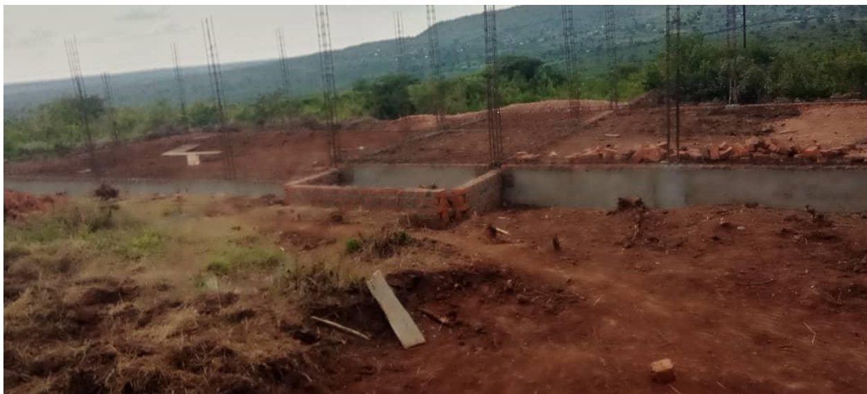
Photographs showing the plinth wall of the dormitory block
