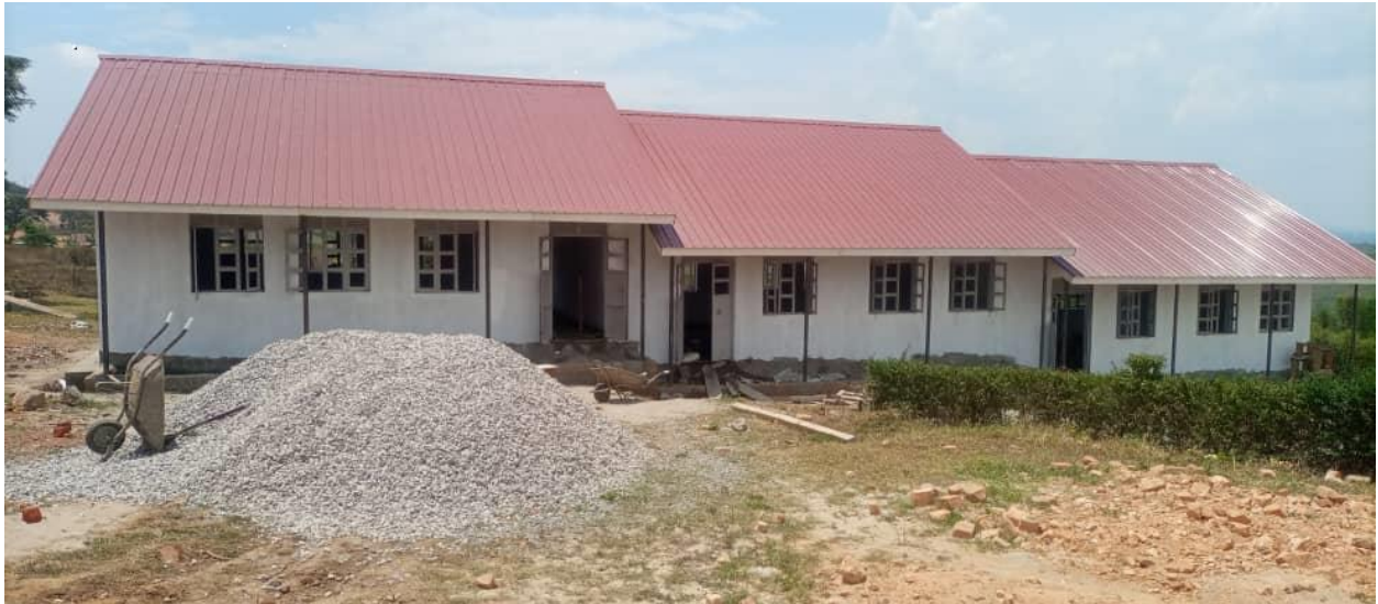
Roof covering for the one unit three classroom block facility
