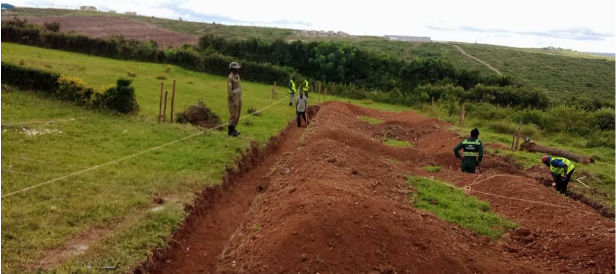
Photograph showing one unit three classroom block foundation excavation
