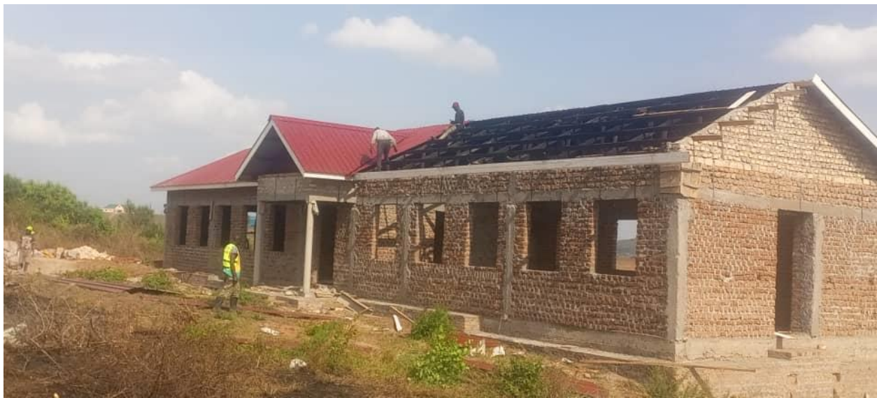
Photographs showing roofing and roof covering for the dormitory block
