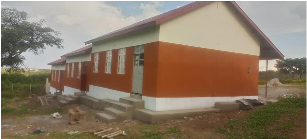
Photograph showing the finished one unit three classroom block facility
