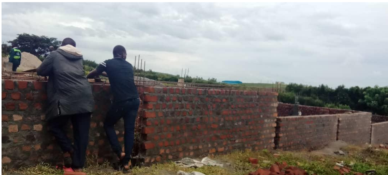
Photographs showing the one unit three classroom block plinth wall construction
