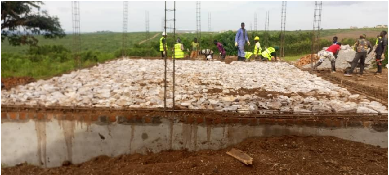
Photograph showing a ground beam and hardcore filling
