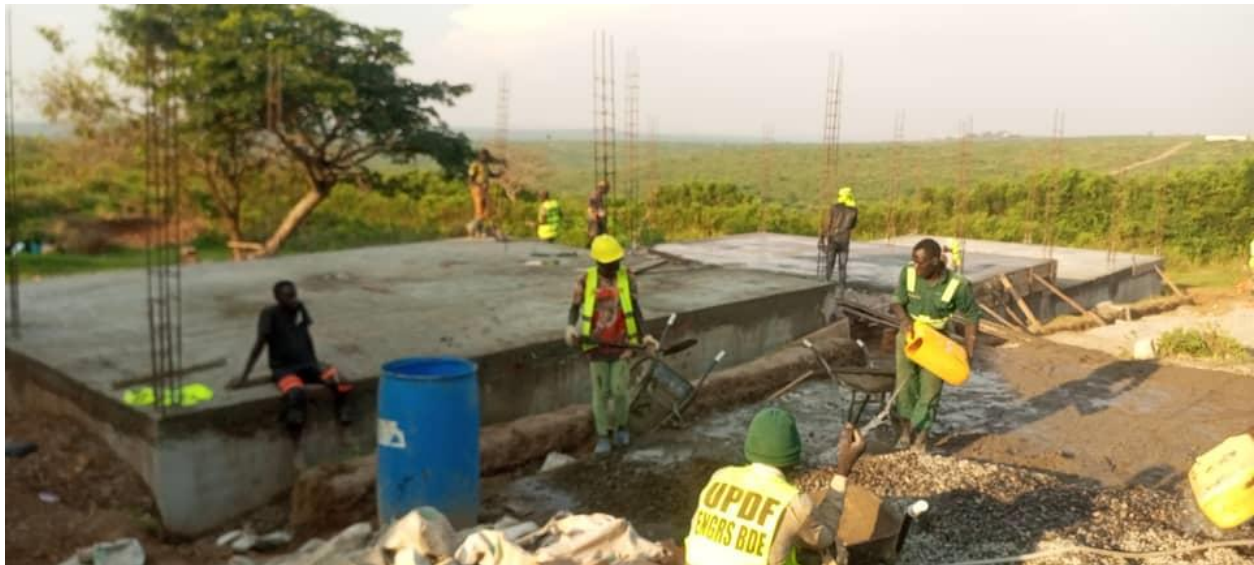
Photograph showing the slab of the one unit three classroom block facility
