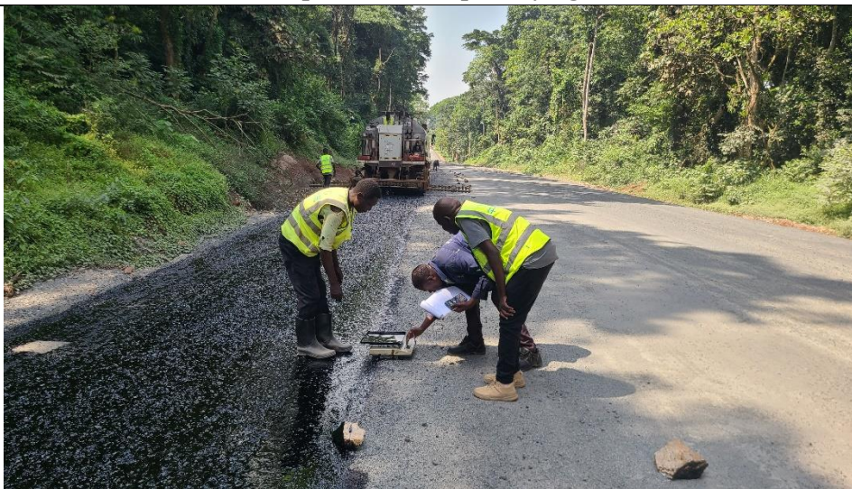
Checking and confirming the spray rate for the bitumen
