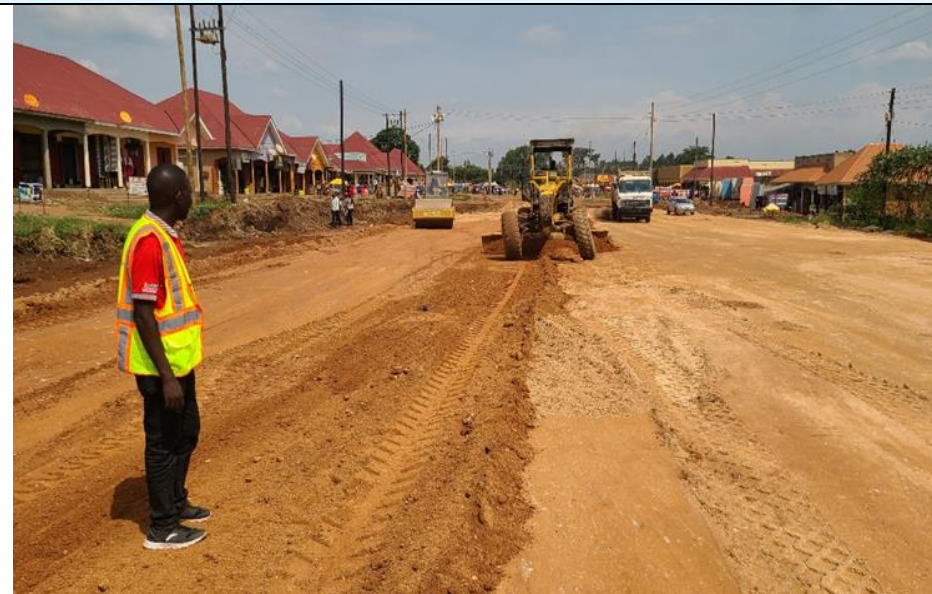
Inspection for G7 3 rd layer fill work at Km 24 F/W town section
