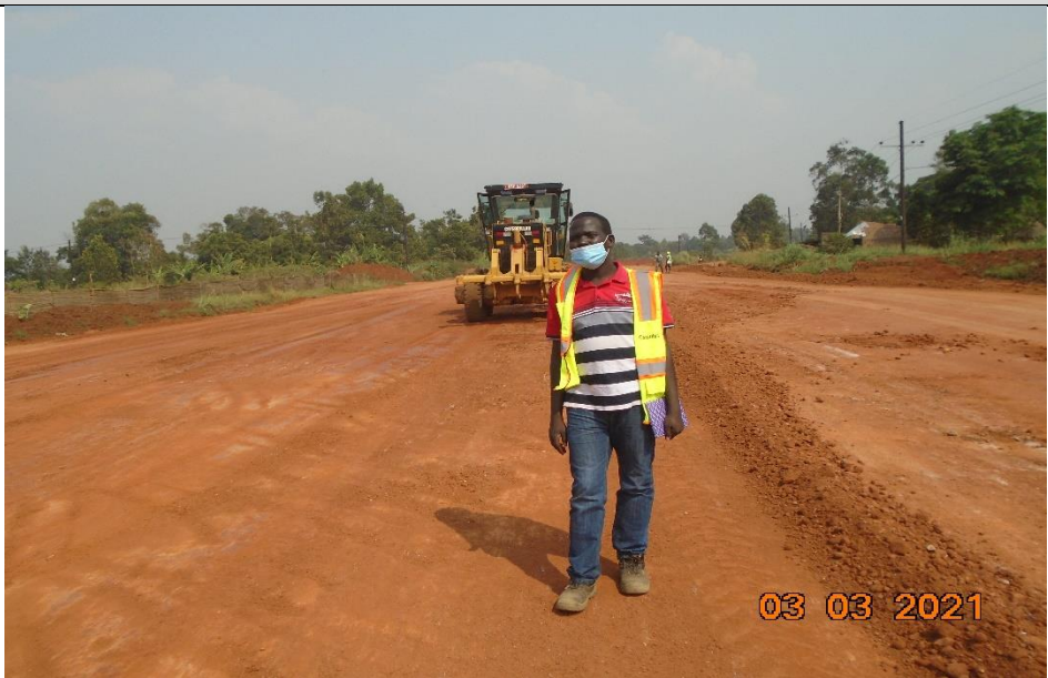
Inspection for G15 top layer
