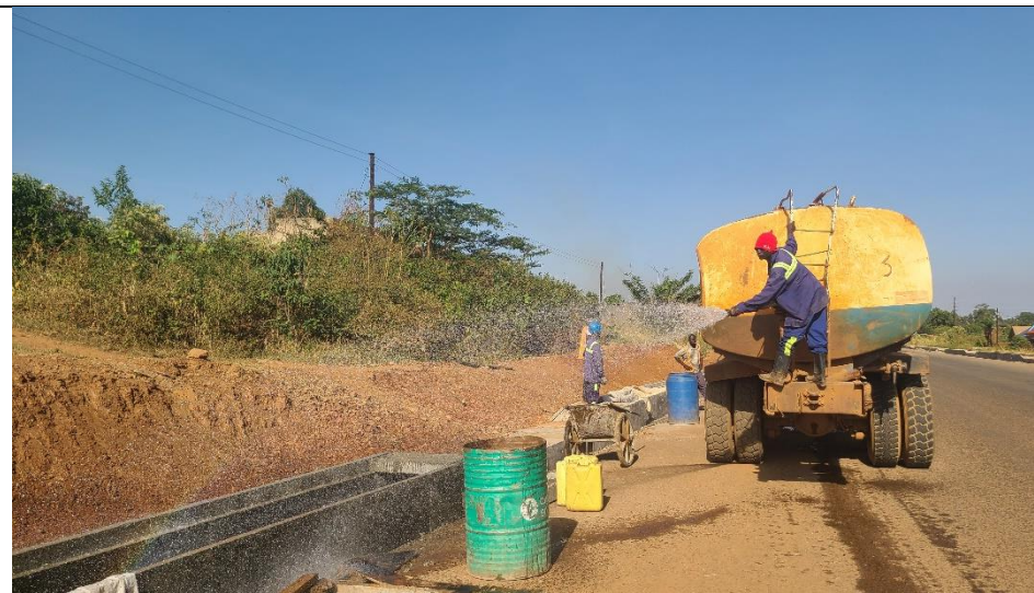
Curing the U-drain
