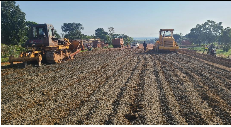
Scarification works for G45 Subbase
