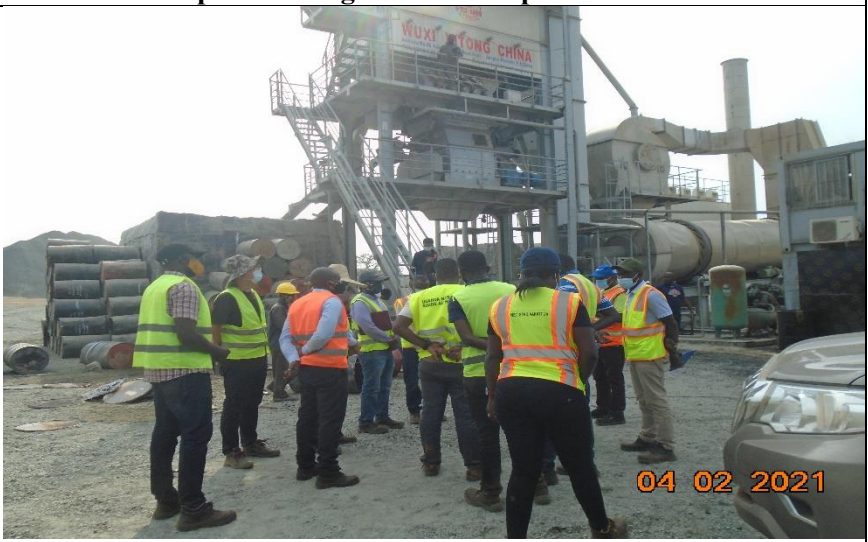
Site Inspection team monitoring the Asphalt plant
