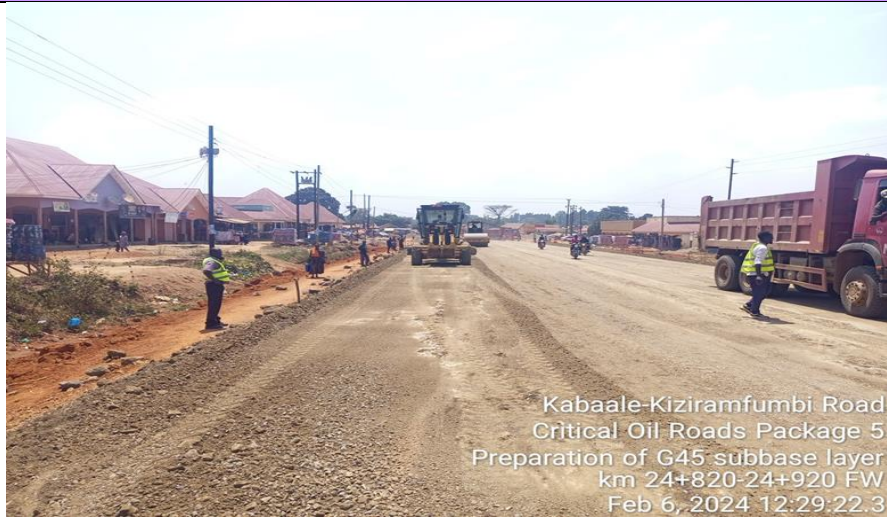
Construction of G45 subbase at Kabaale Town
