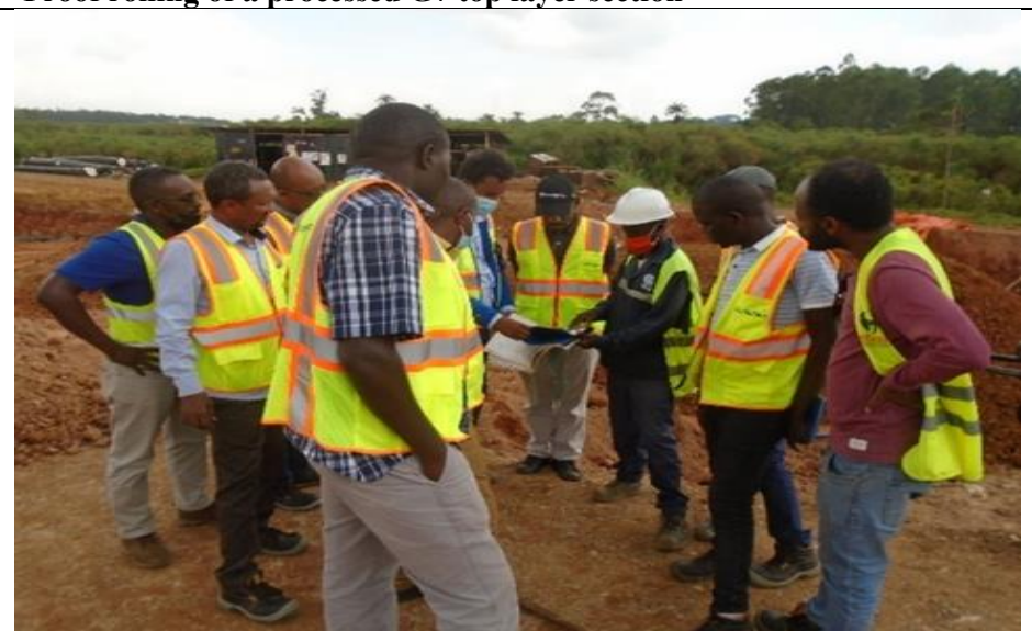
Photo showing the Monthly Site Inspection
