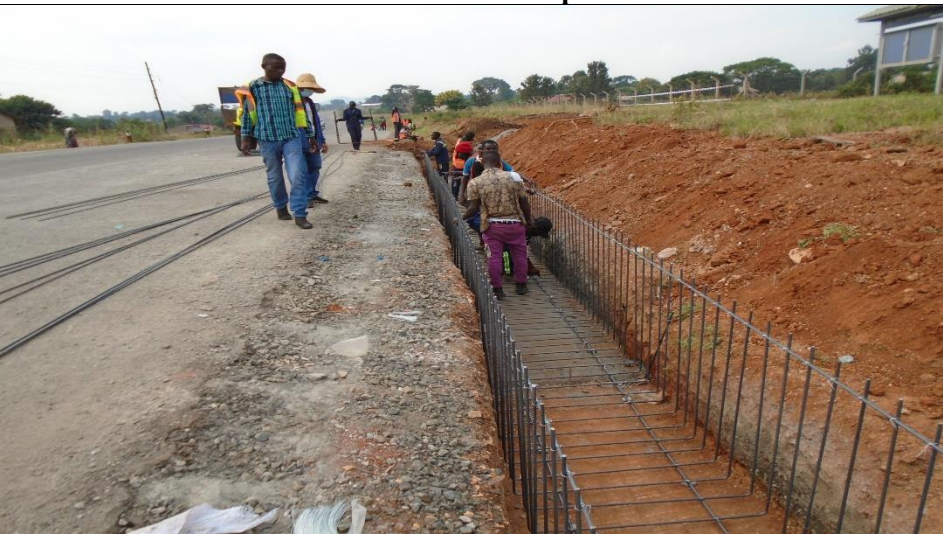
Inspection for the U-drain steel reinforcement along KK road
