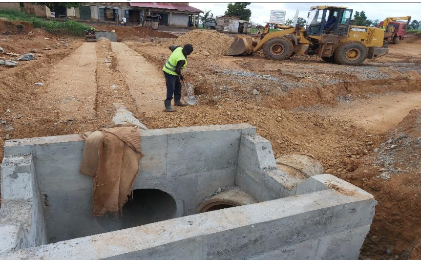
Pipe Culvert backfill along KK road
