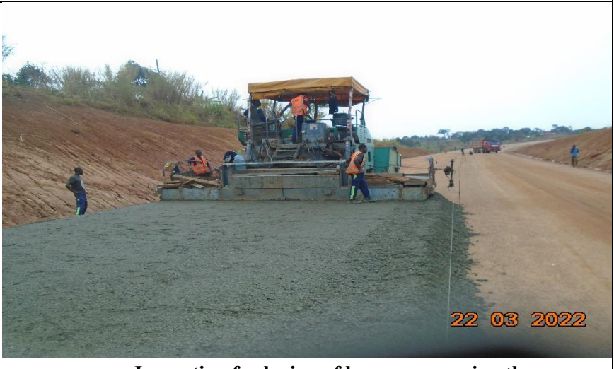
Inspection for laying of base course using the paver
