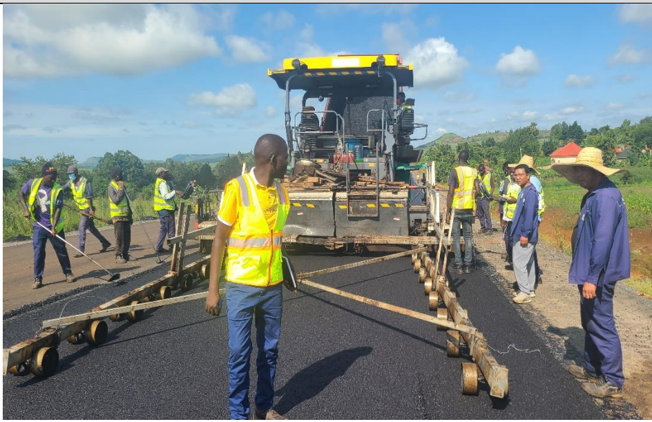
Inspection for Aspalt laying
