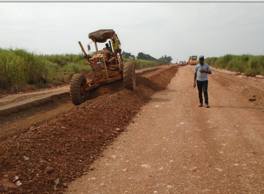
Inspection for the bench-works for G45 subbase
