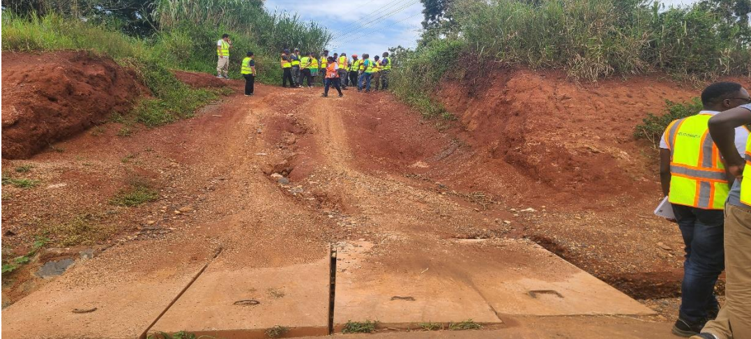
Crossing slabs provided for Homesteads along KK road
