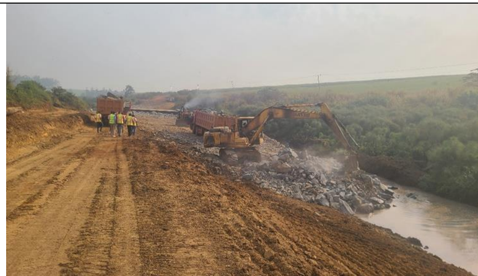
Inspection for rock fill (swamp treatment) at Km 17LHS
