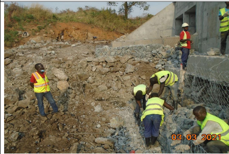
Inspection for gabion box works at the Box Culvert End Structures
