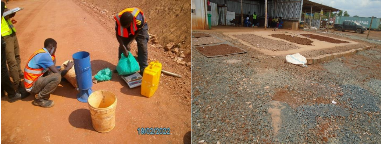
Photos showing field density test and Material drying for CBR determination
