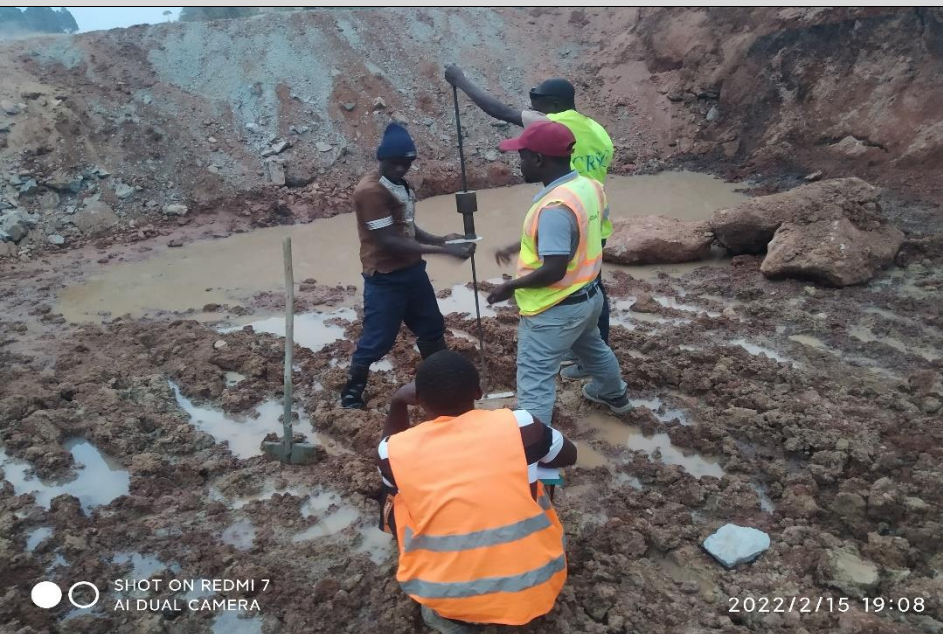
DCP works at the swamp section
