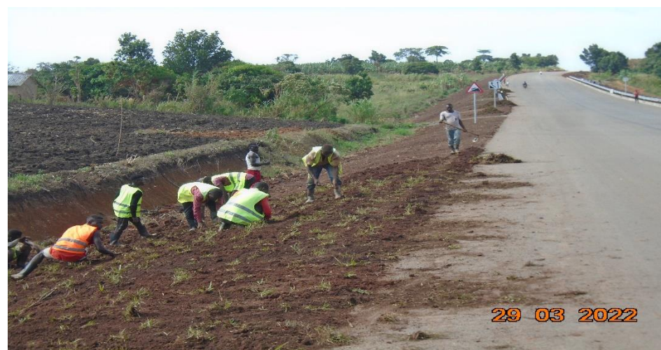
Inspection for grassing for landscape along the high fill section
