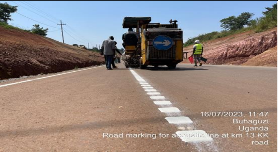
Road marking along Kabaale-Kiziranfumbi road
