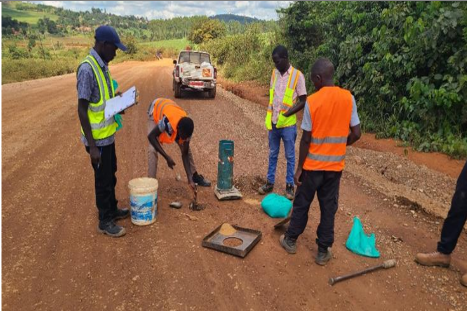
Field Density Test by san replacent
