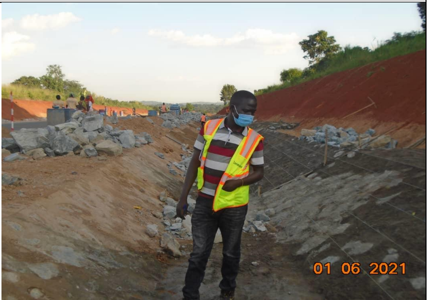
Inspection for grouted stone-pitched works
