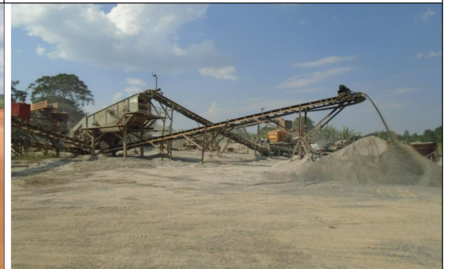
Monitoring wet crushing at the quarry
