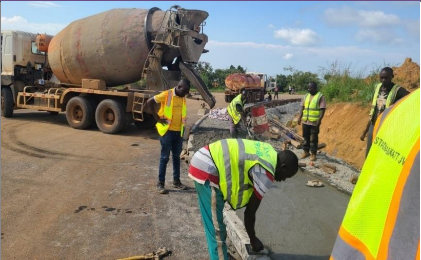
Casting Concrete for walkways
