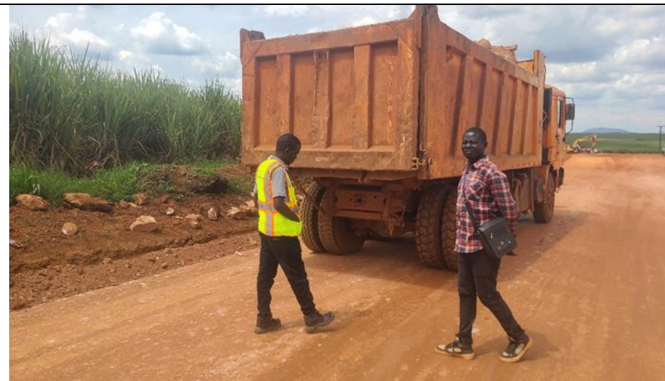
Proof rolling of a processed G7 top layer section
