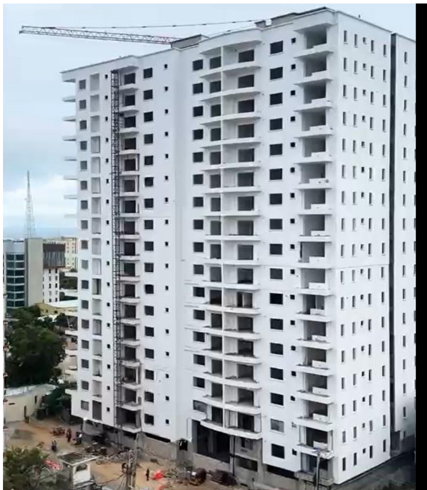
Figure 14: Entire building structure
