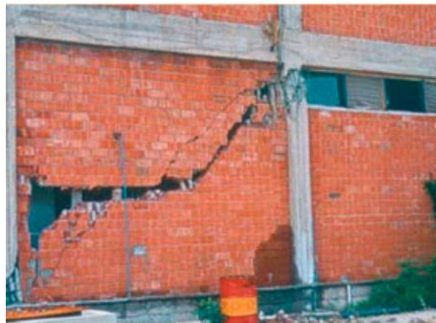
Figure 2.3 Diagonal Cracking
