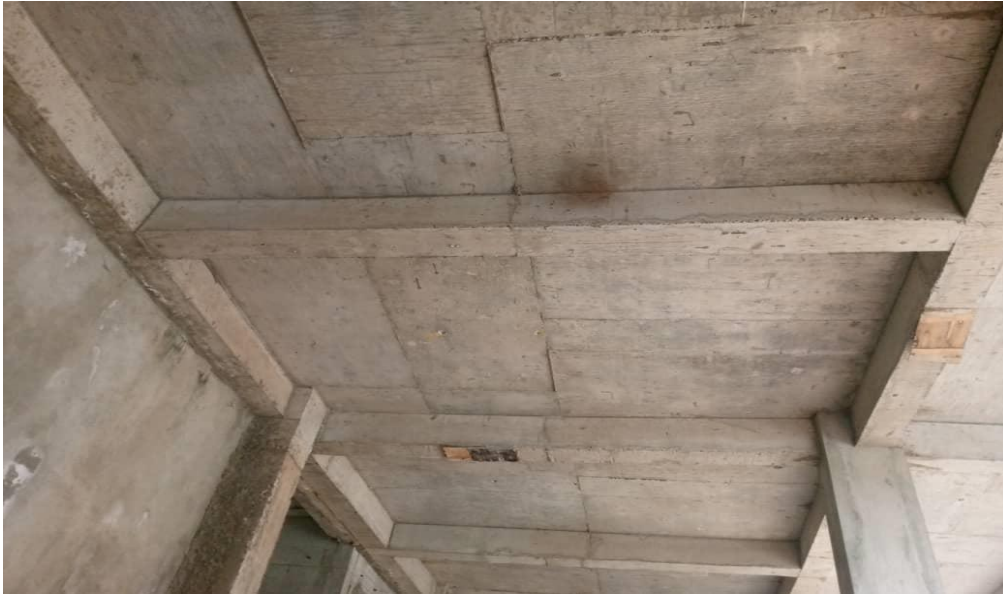
Figure A 10. A photo showing the soffits of an RCC slab
