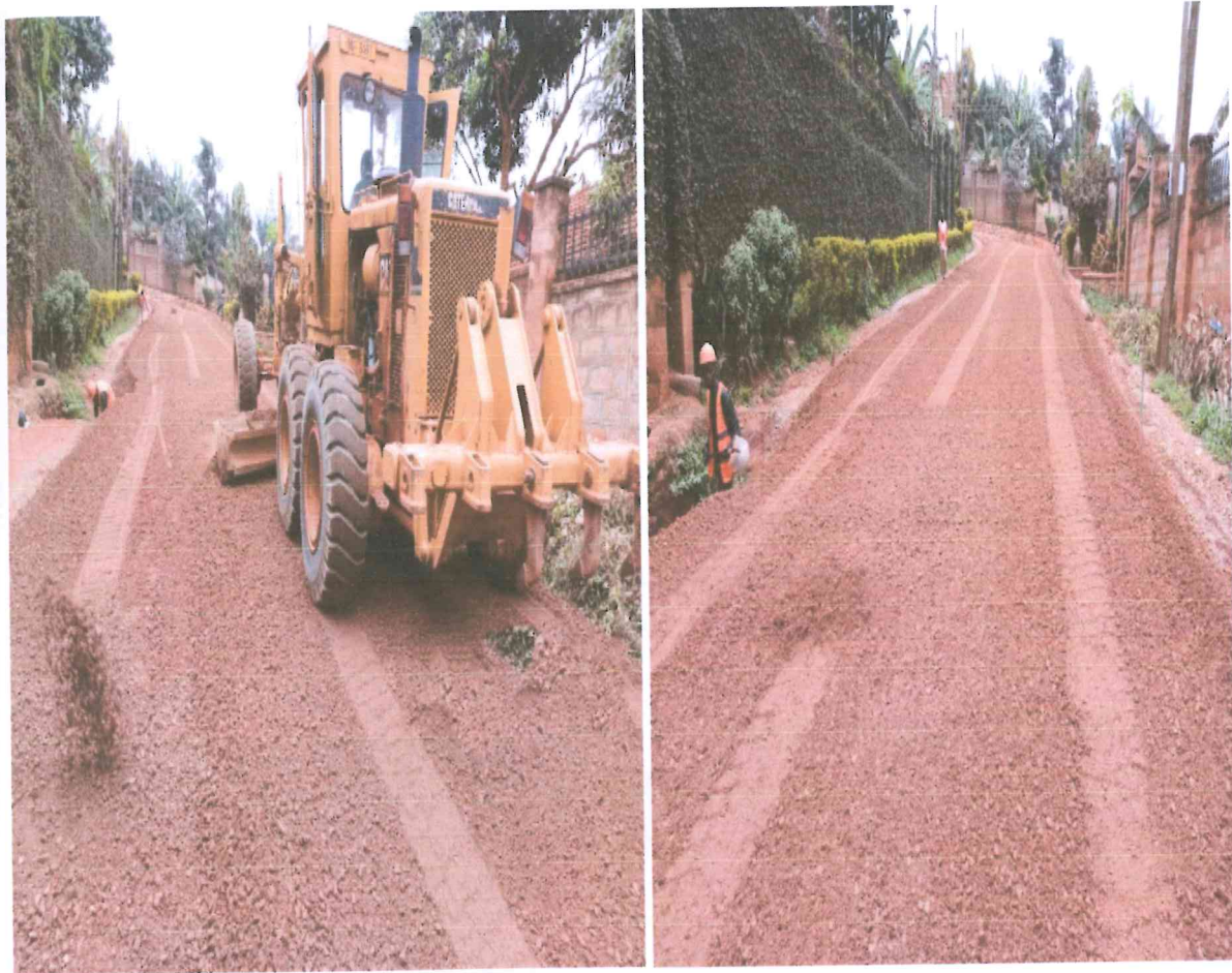
Figure 2:11 Construction of the base layer
