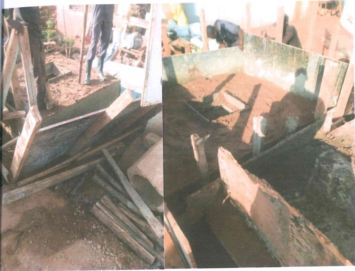
Figure 2:6 Formwork on a manhole
