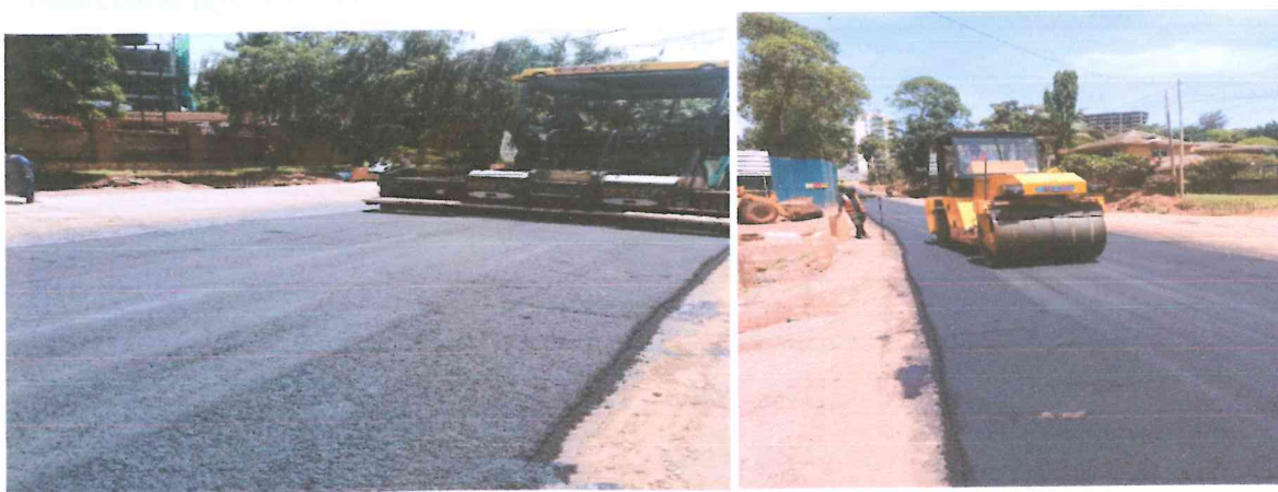
Figure 2:12 Laying and compaction of asphalt
