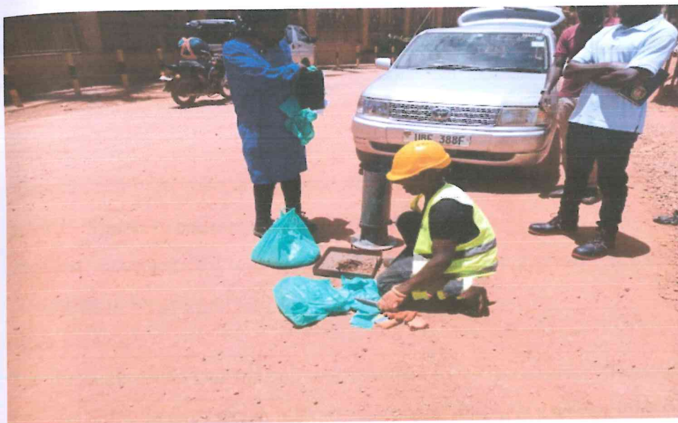
Figure 2:13 Testing of the sub base layer
