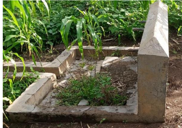
One of the broken taps in the settlement
