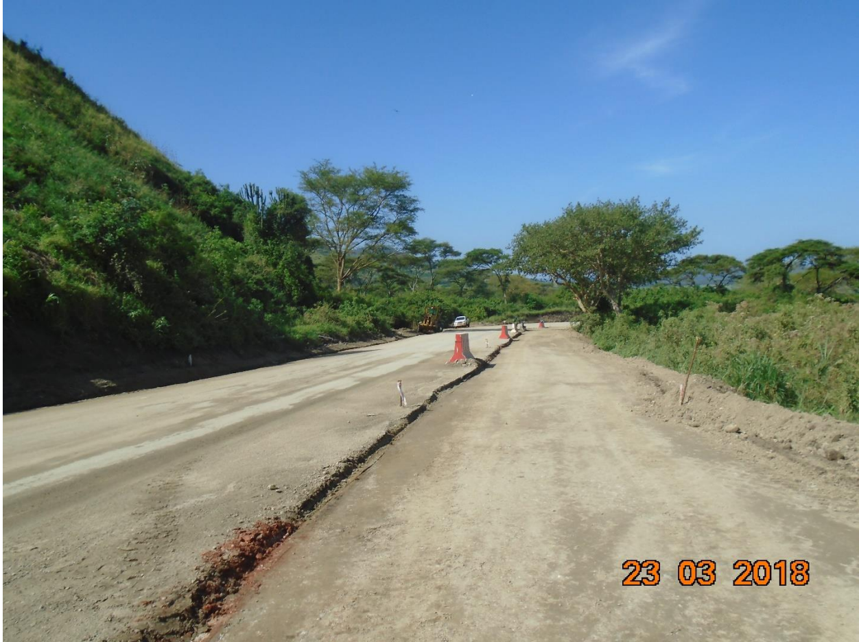
Figure 10 A well compacted sublayer Section of the road
