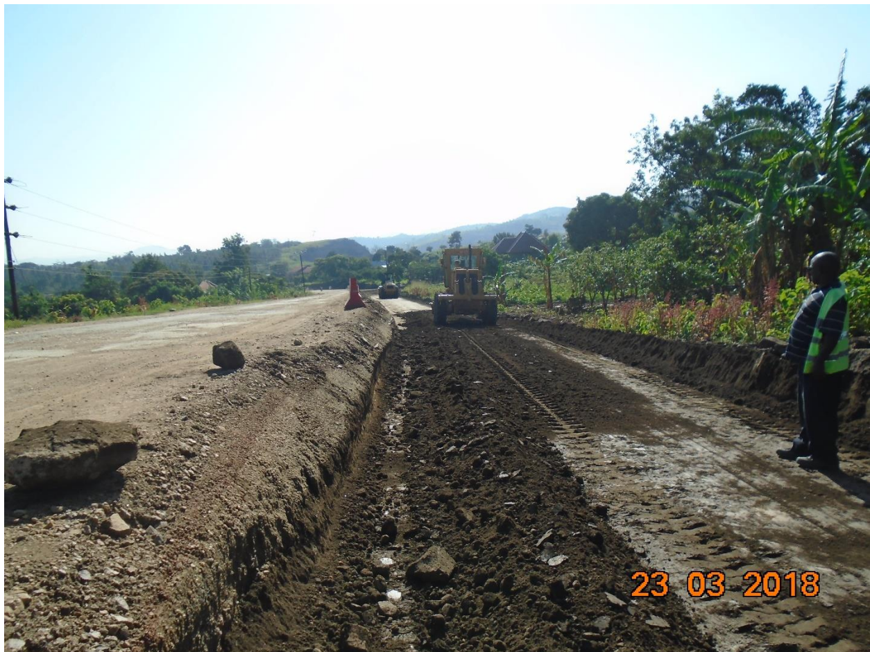
Figure 8 Roadbed Preparation
