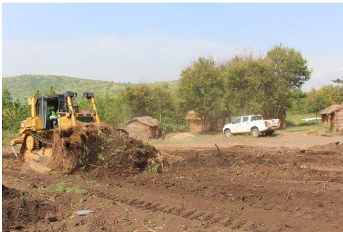
Figure 6 Clearing and Grubbing works using a D6 Dozer
