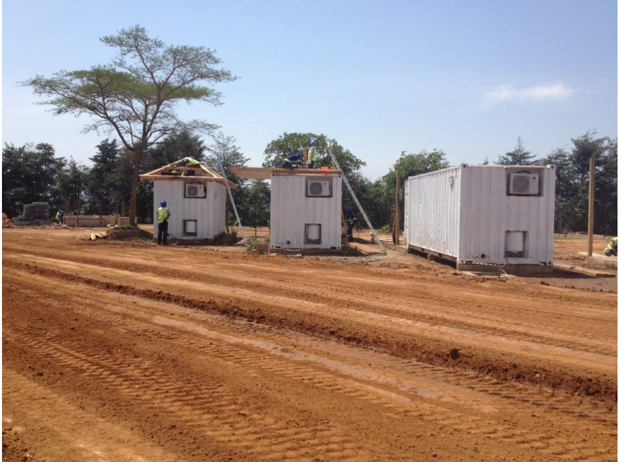
Figure 2 Site Camp Establishment Works
