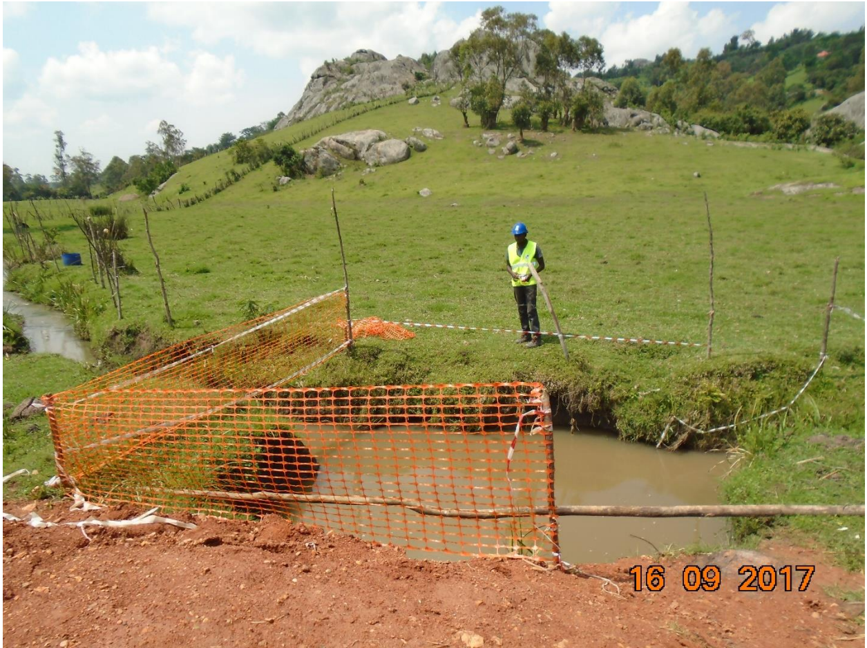
Figure 14 Environmental Protection at the Quarry
