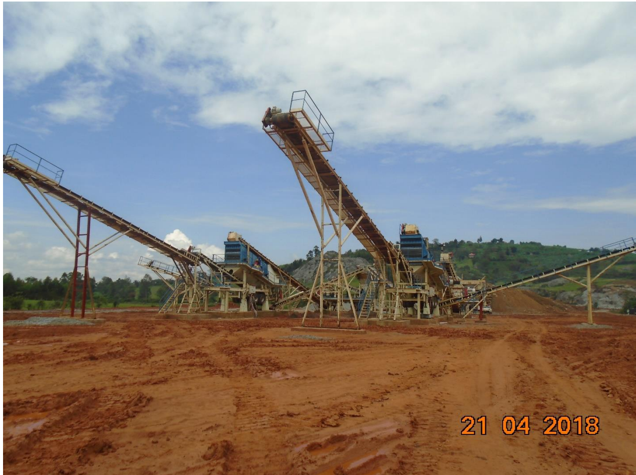
Figure 3 Rock Quarry Establishment works
