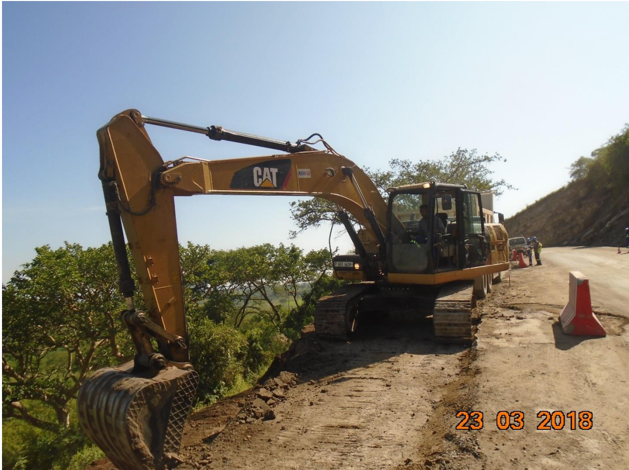
Figure 7 Clearing on the slopes
