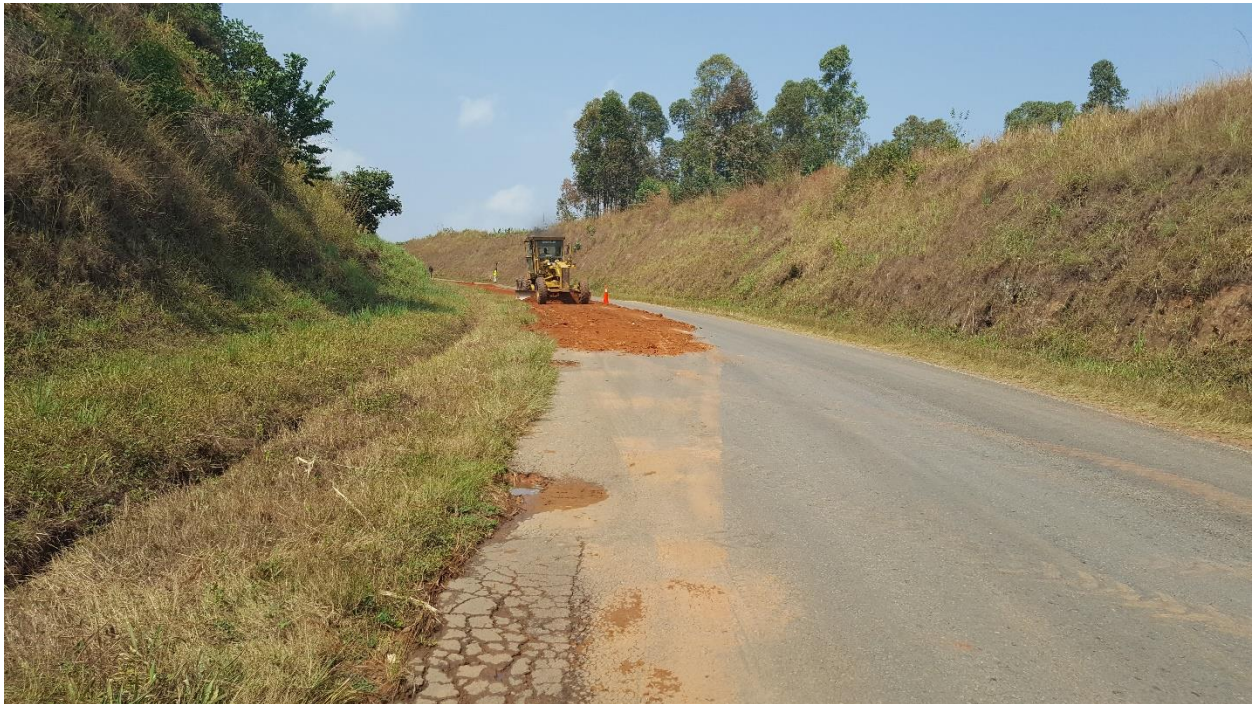
Figure 5 Wheel Loader correcting a section during Forward Maintenance Works
