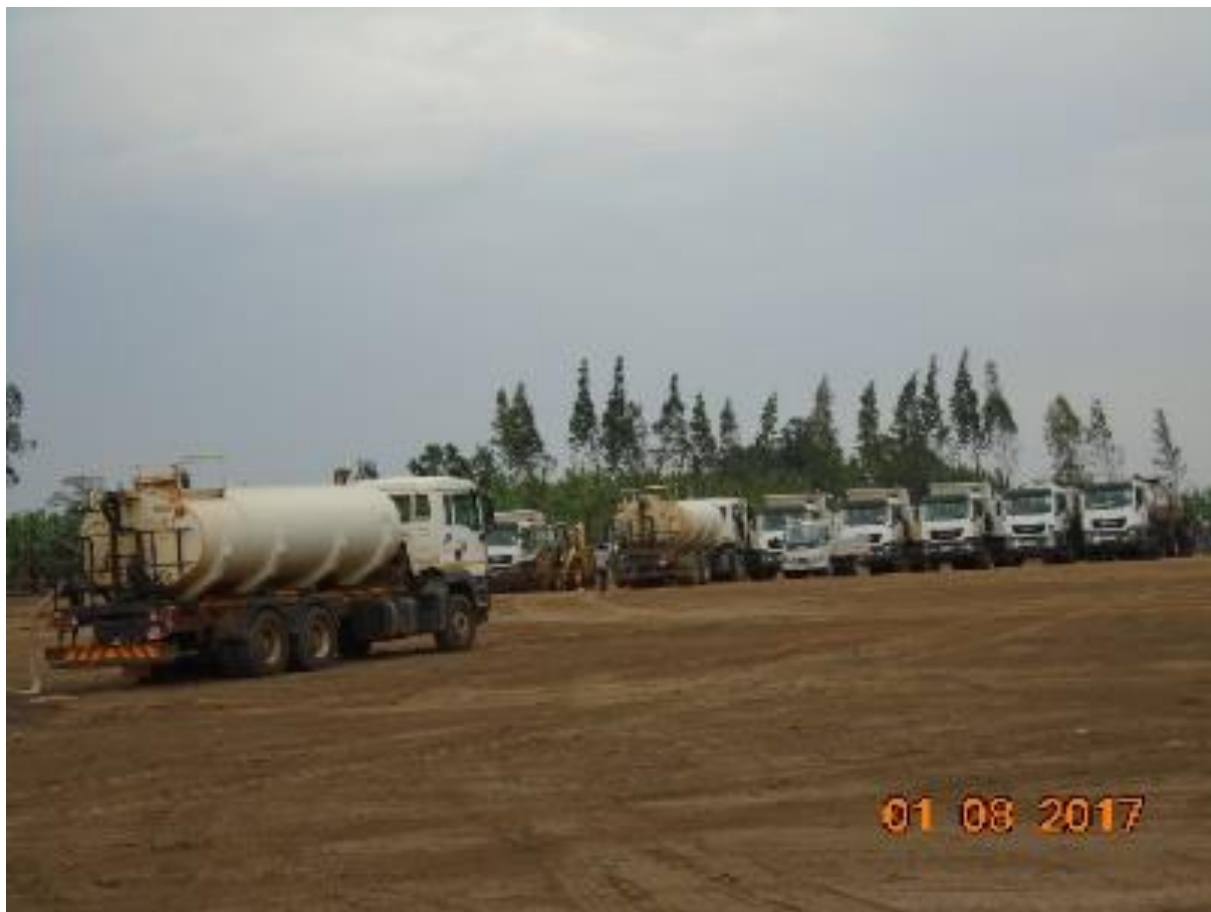
Figure 4 Some of the Equipment Mobilised at Commencement
