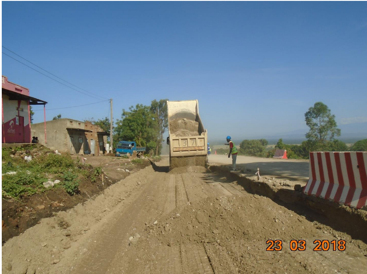
Figure 9 Dumping of Borrow material (G15) during sublayer formation
