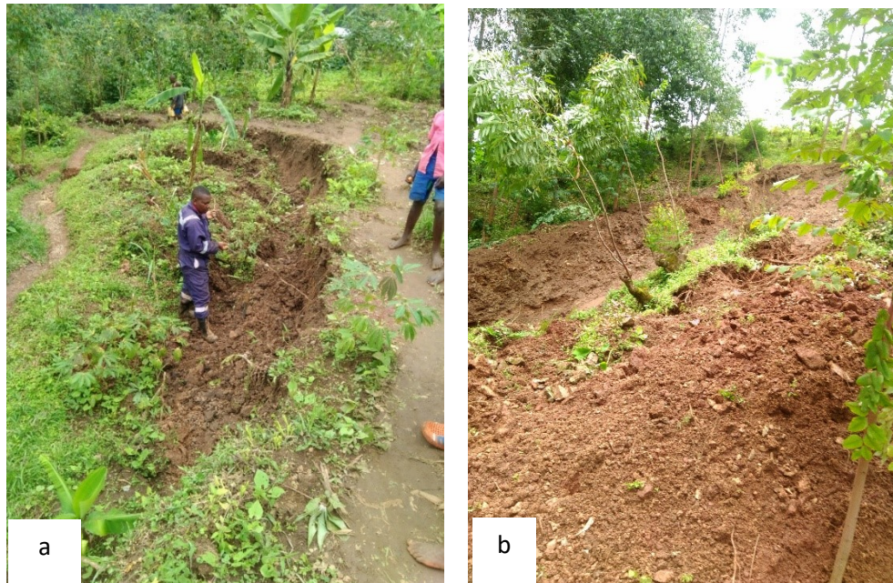
Figure 1: Landslide cracks in Nakhatore village, Tsume micro-catchment
